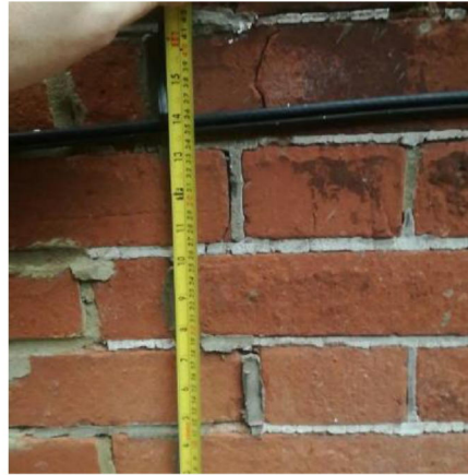
Damage outside kitchen, note the previous repairs
