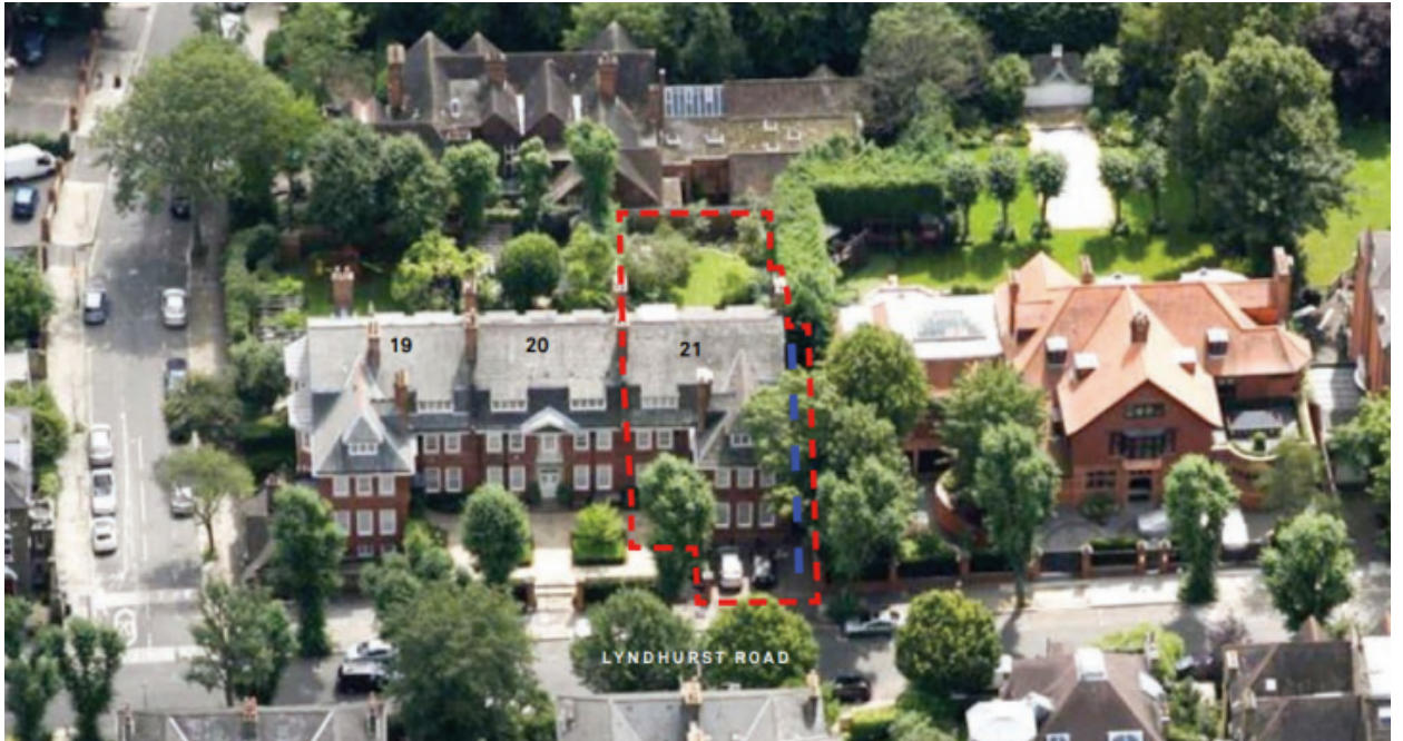
Figure 1: Google Aerial Image of 21 Lyndhurst Road
