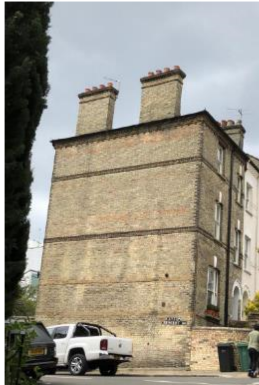
#View of side of property
