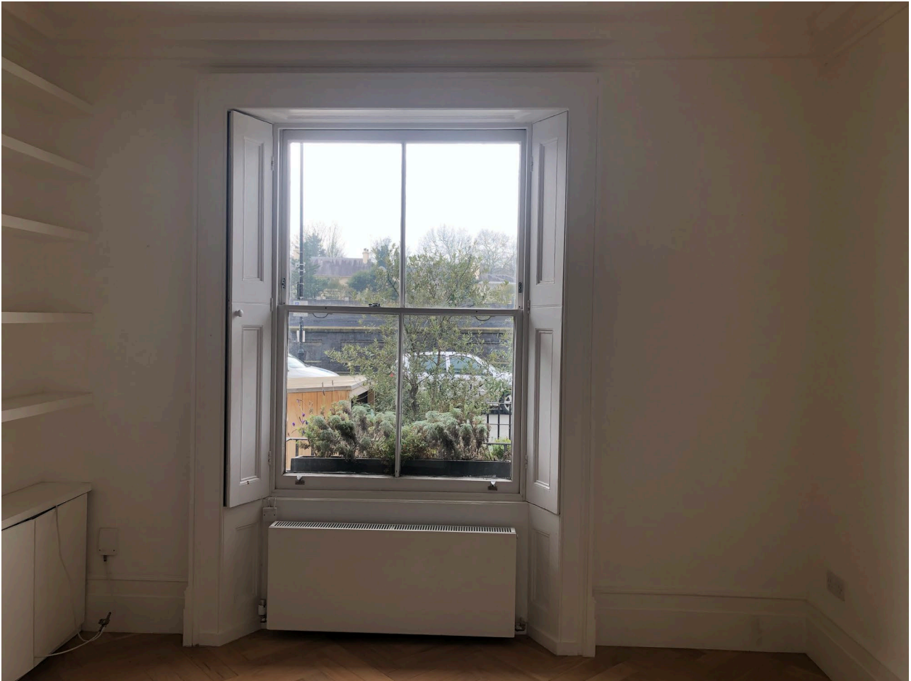
Figure 5: Internal view of the front external wall at ground floor
