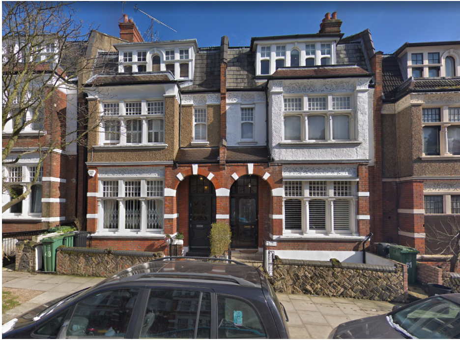
Photo 1 (above): front elevation (application site on left)
