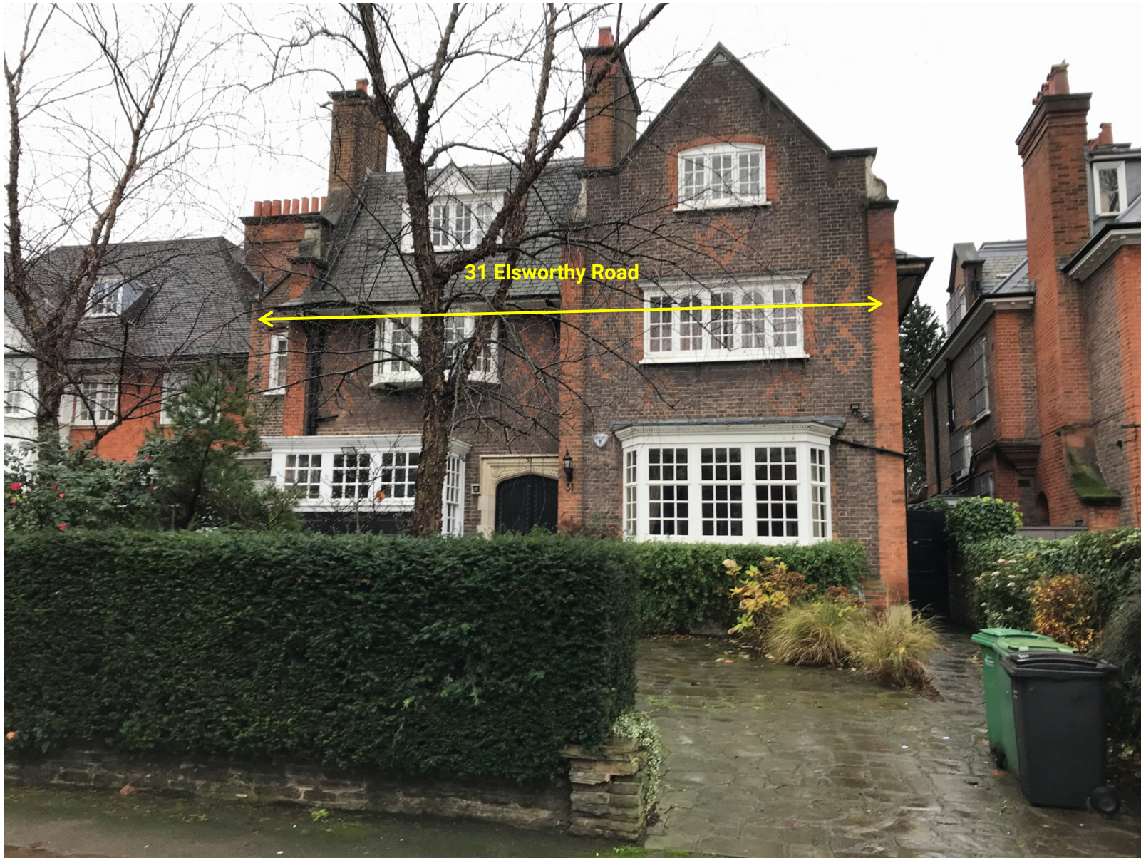
Photo A: View of front façade of property at 31 Elsworthy Road, London NW3
