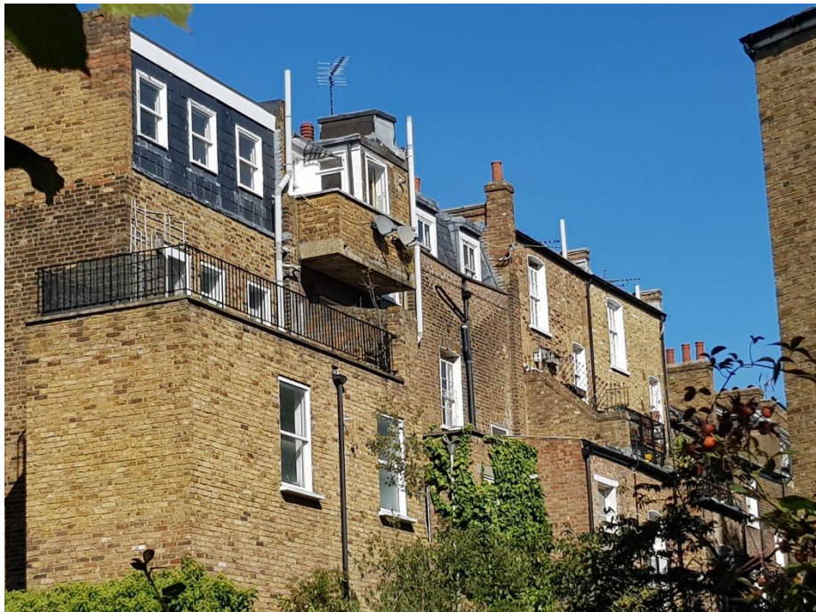
View of the existing rear of the property
