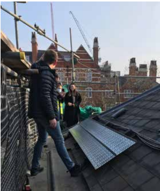
Mock up of electrical containment location and impact on roof
