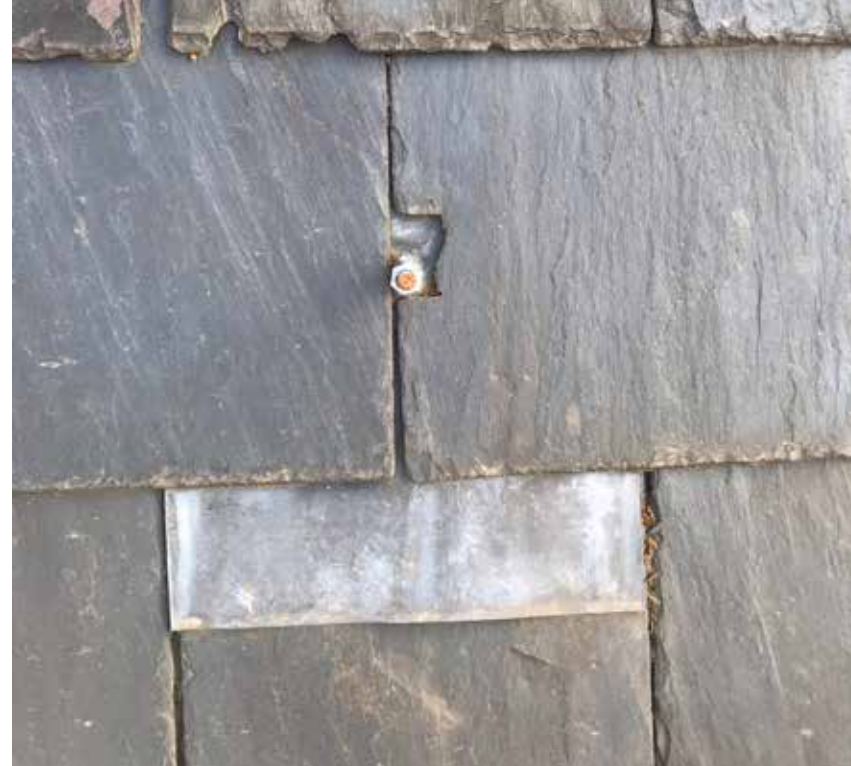
Penetration detail as consented for safety cable anchorage for mansafe system
