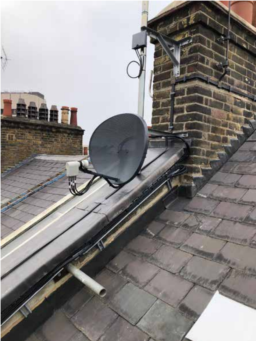
Lowered to sit against the lead covered coping
