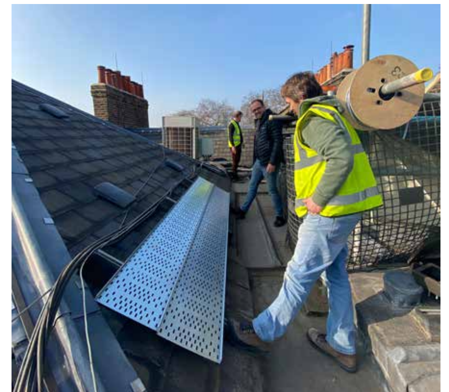
Mock up of electrical containment location and impact on roof
