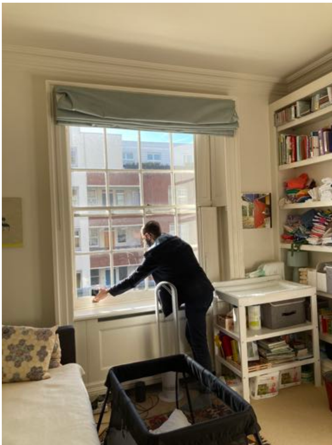
Second floor rear bedroom window with original architrave and shutters in part.
