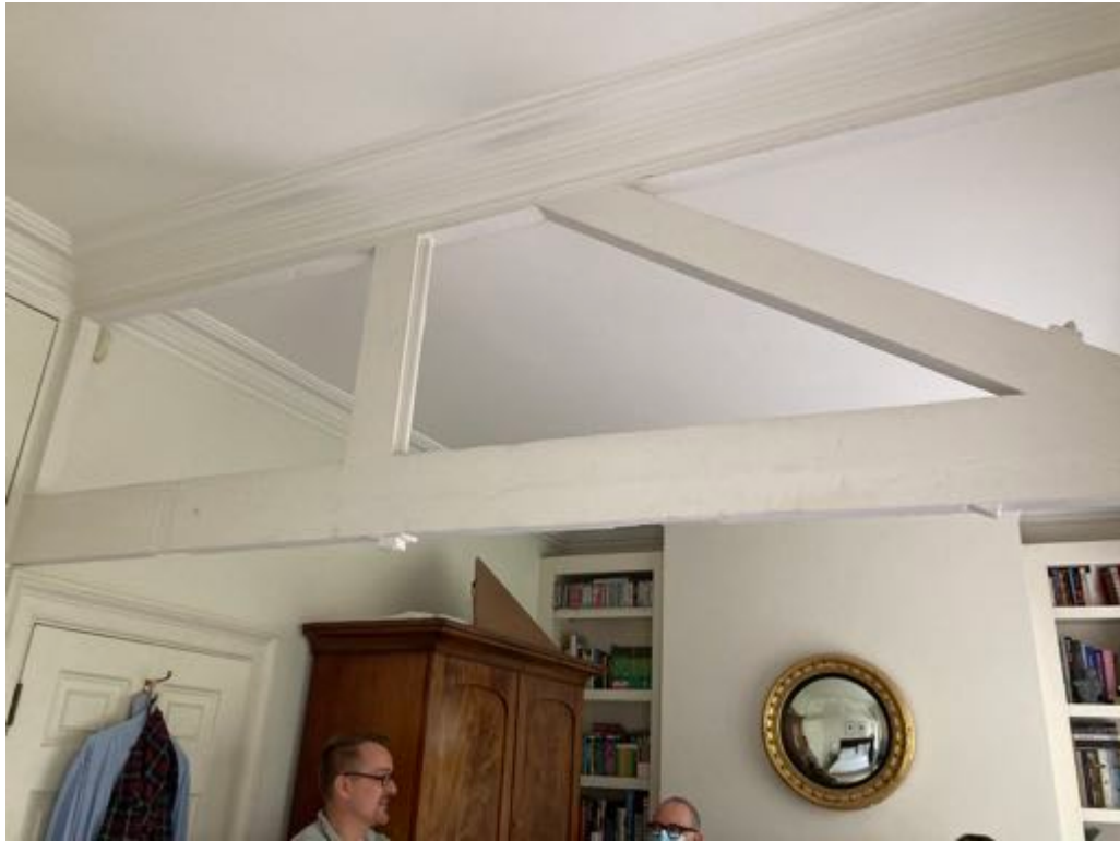
Second floor front bedroom wall truss.
