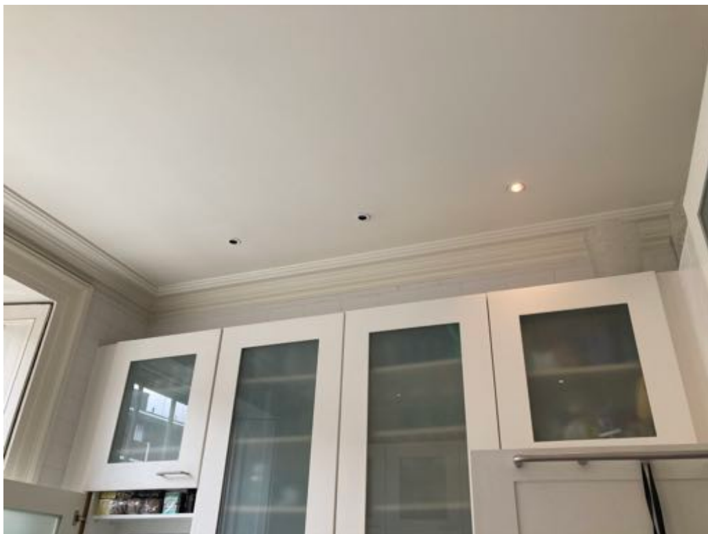
The kitchen has false walls and a lowered ceiling with modern cornice. The window architrave appears original.
