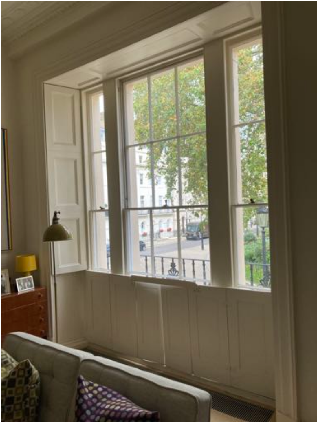
First floor front. Shutters are a combination of old and new elements. The central sash is modern but the margin lights appear to be original.
