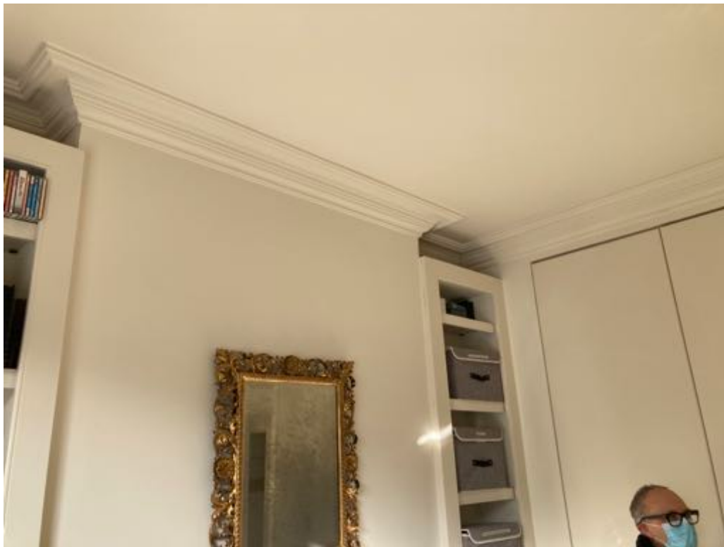
Modern cornicing runs around the modern partitions.
