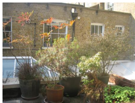
Above: View at ground floor level across rooflight towards kitchen windows of 54 Cumberland Terrace/28 Cumberland Terrace Mews.
