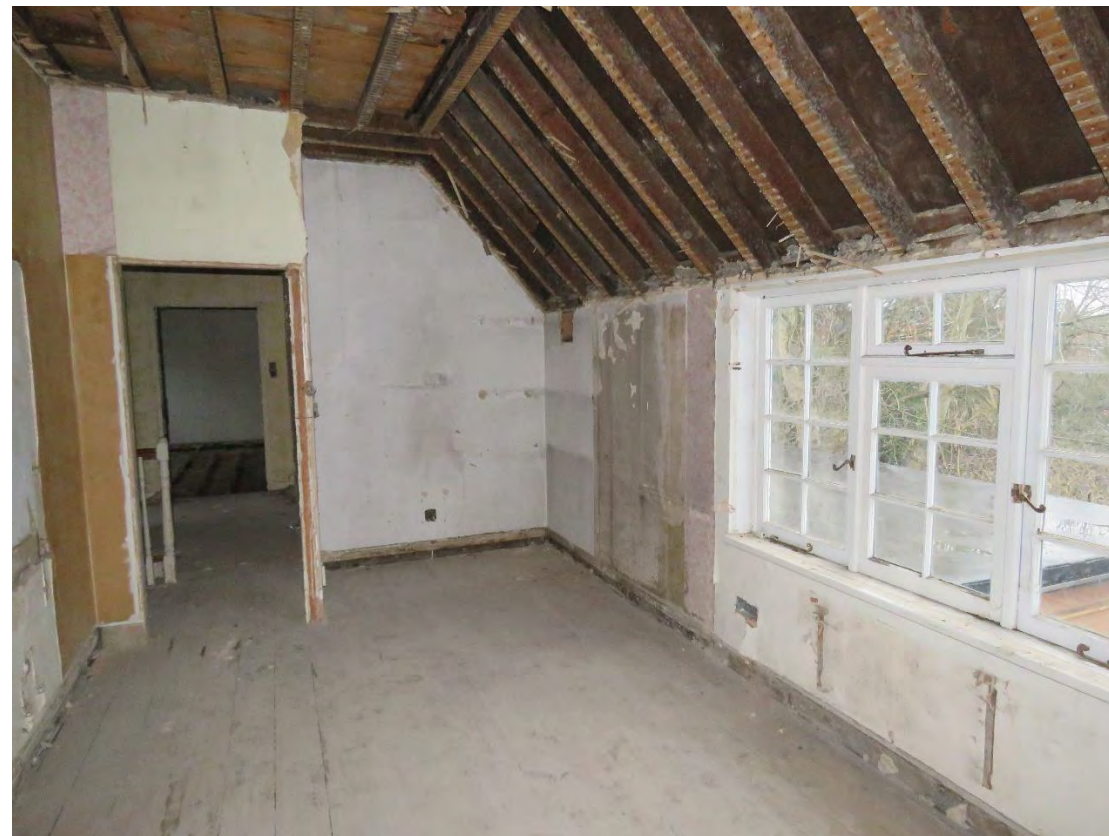
Figure 46: View looking north towards the stair landing. Note the modern studwork partition wall with the door opening. The c.1960s windows are seen to the right.
