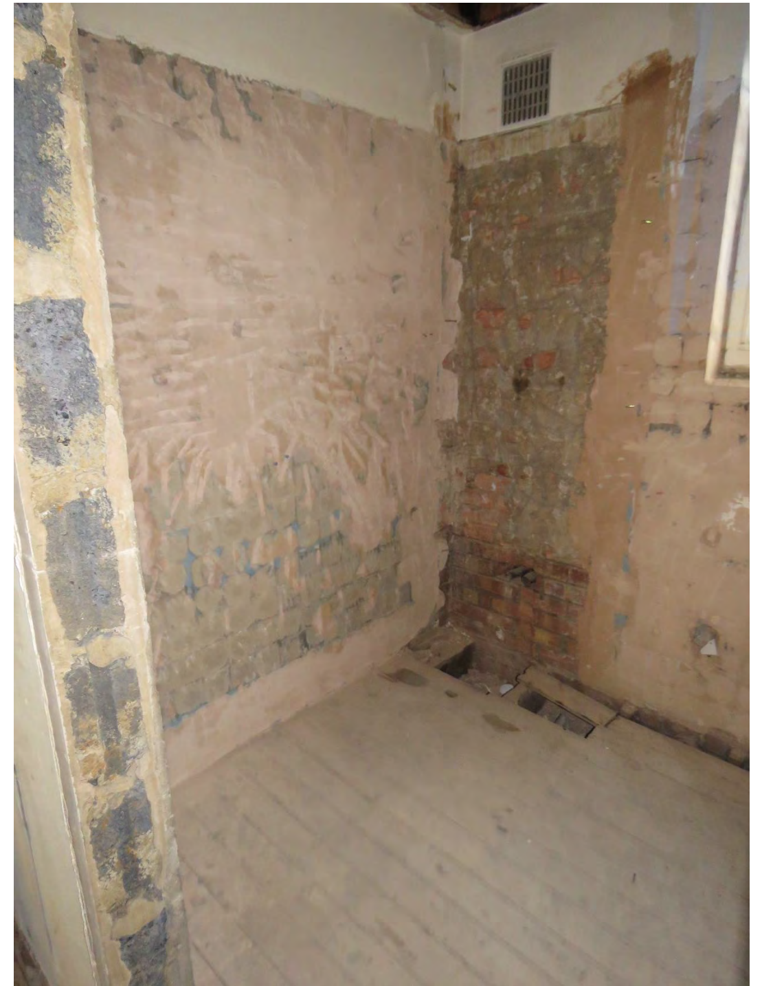
Figure 55: View of the WC/ shower area, part of the dressing room (south side). Note the concrete block partition walls and non-original wall and floor finishes.
