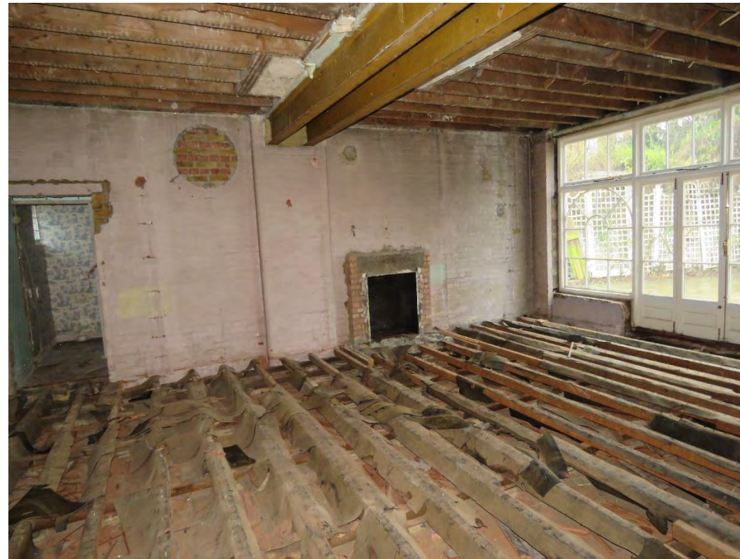
Figure 22: View of the reception room, looking south. Note the later 'fireplace' on the south wall, blocked bulls eye window. The steel I sections spanning the room and supporting the timber joists may be a later intervention necessitated by intrusive structural works in this area. The conservatory style glazed French doors to the right are modern.
