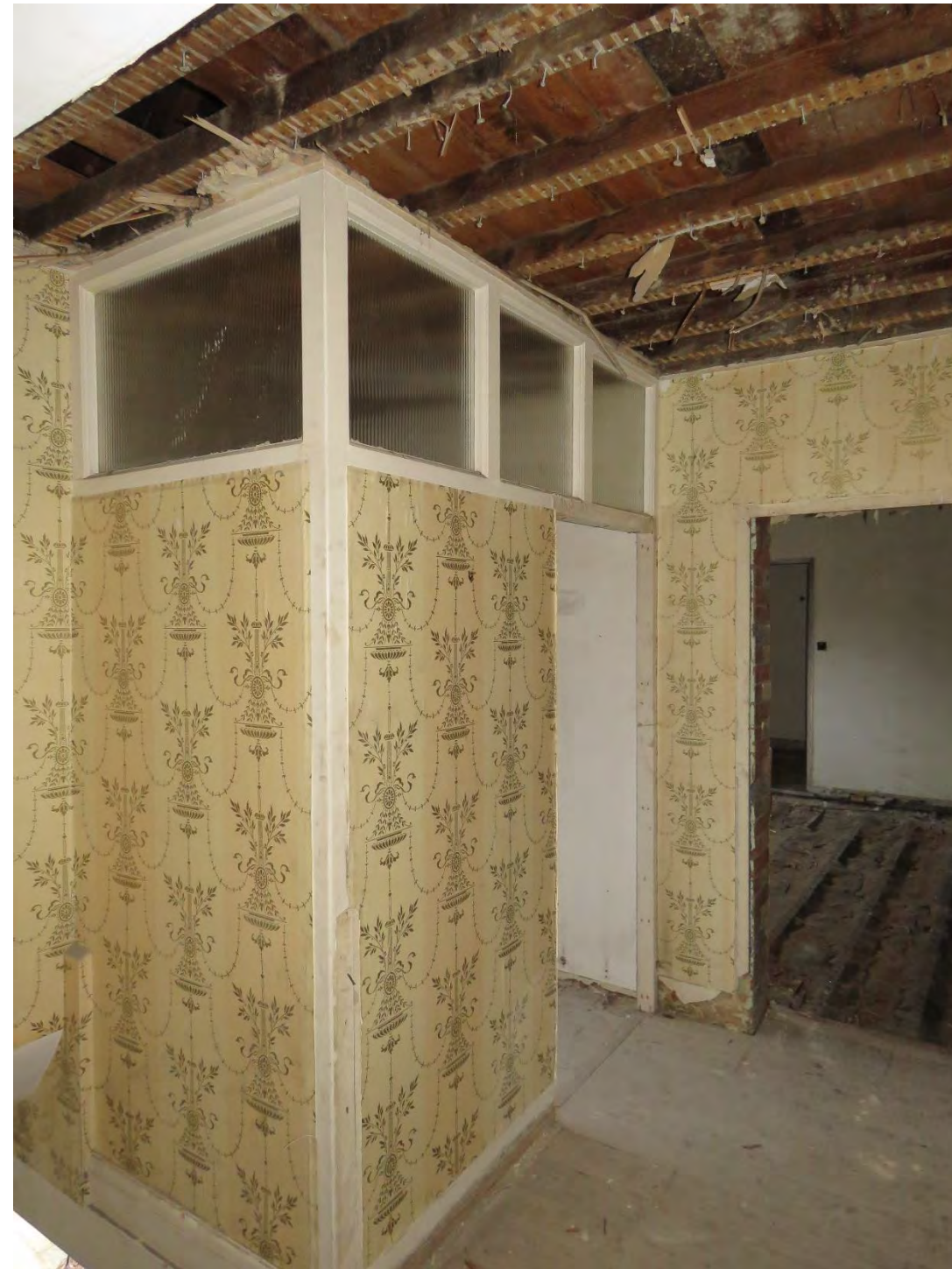
Figure 38: The modern enclosure at first floor. The enclosure is built with studwork partition walls and has glazed sections above. This view looks towards the bedroom to the north. A view of the inside of this enclosure is included in Figure 40
