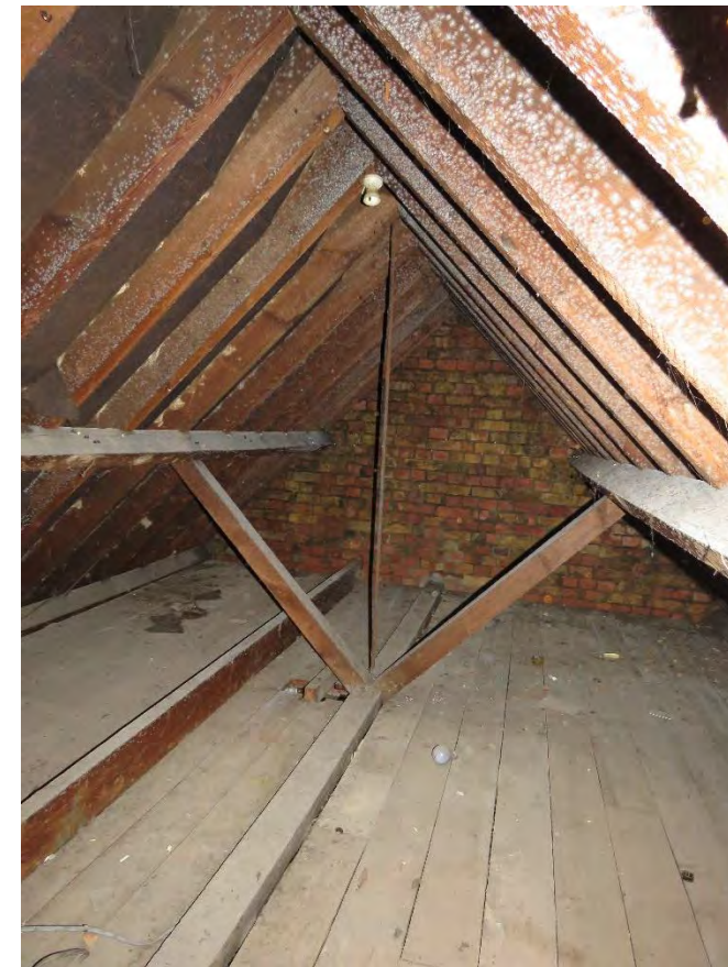
Figure 71: View of the cut roof construction towards the west (front) elevation.
