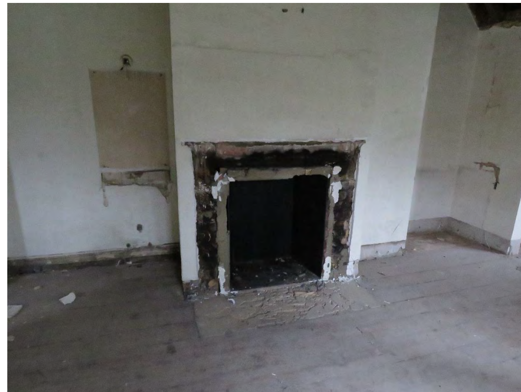
Figure 42: Close up view of the chimney breast showing the location of the fireplace (removed).
