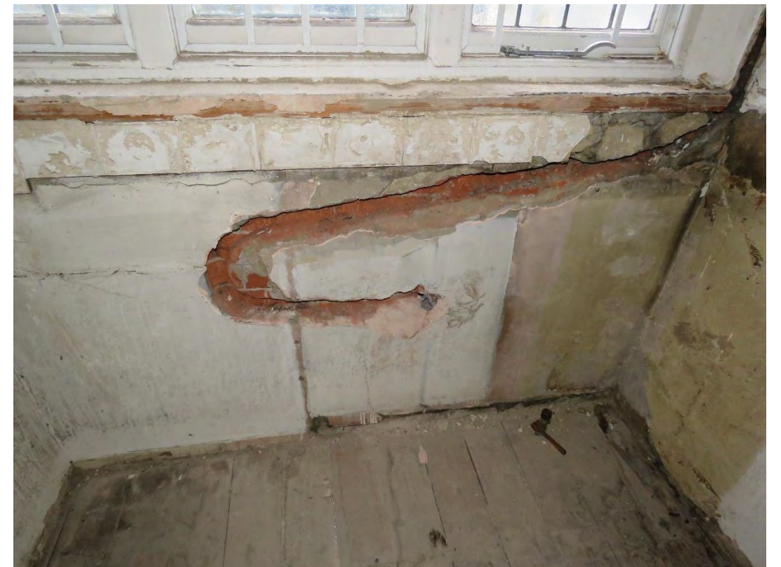
Figure 40: View of the west wall of the enclosure showing the original brick wall with chased plumbing (removed) and part of the windows. This area preserves no original finishes or details.
