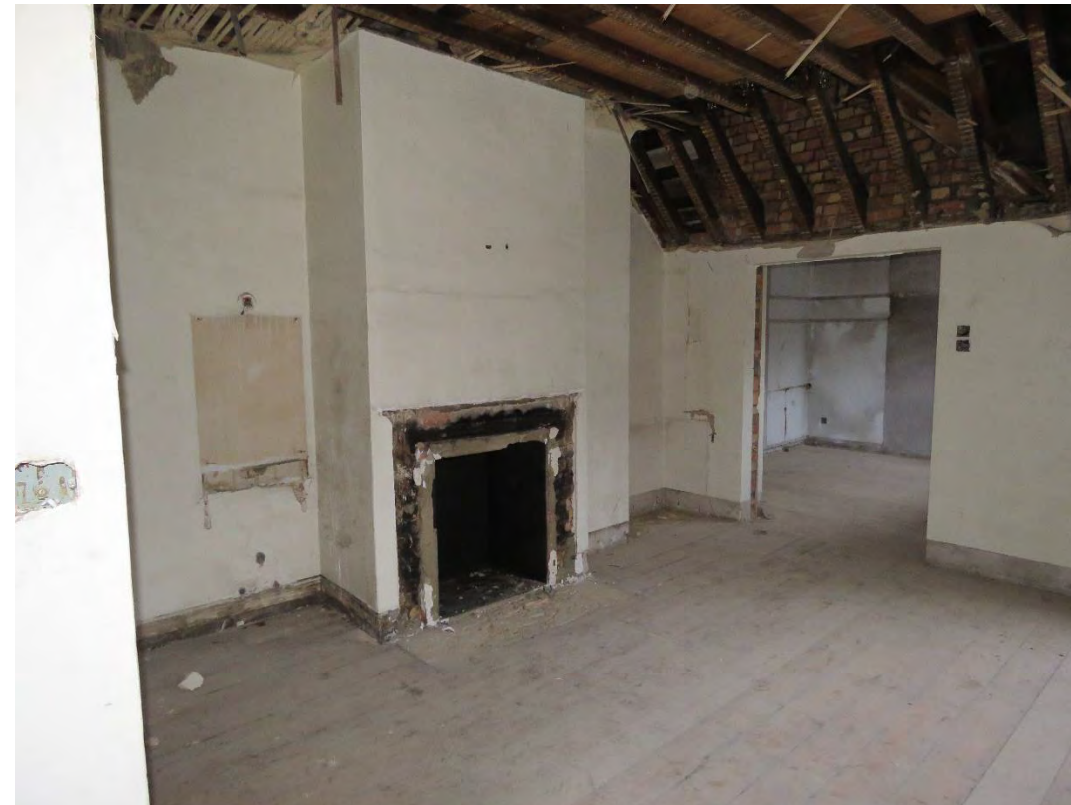
Figure 41: View of Bedroom 1 showing the chimney breast. Note the altered opening in the background. Some floorboards in this room appear to have been altered when the north wall was changed.
