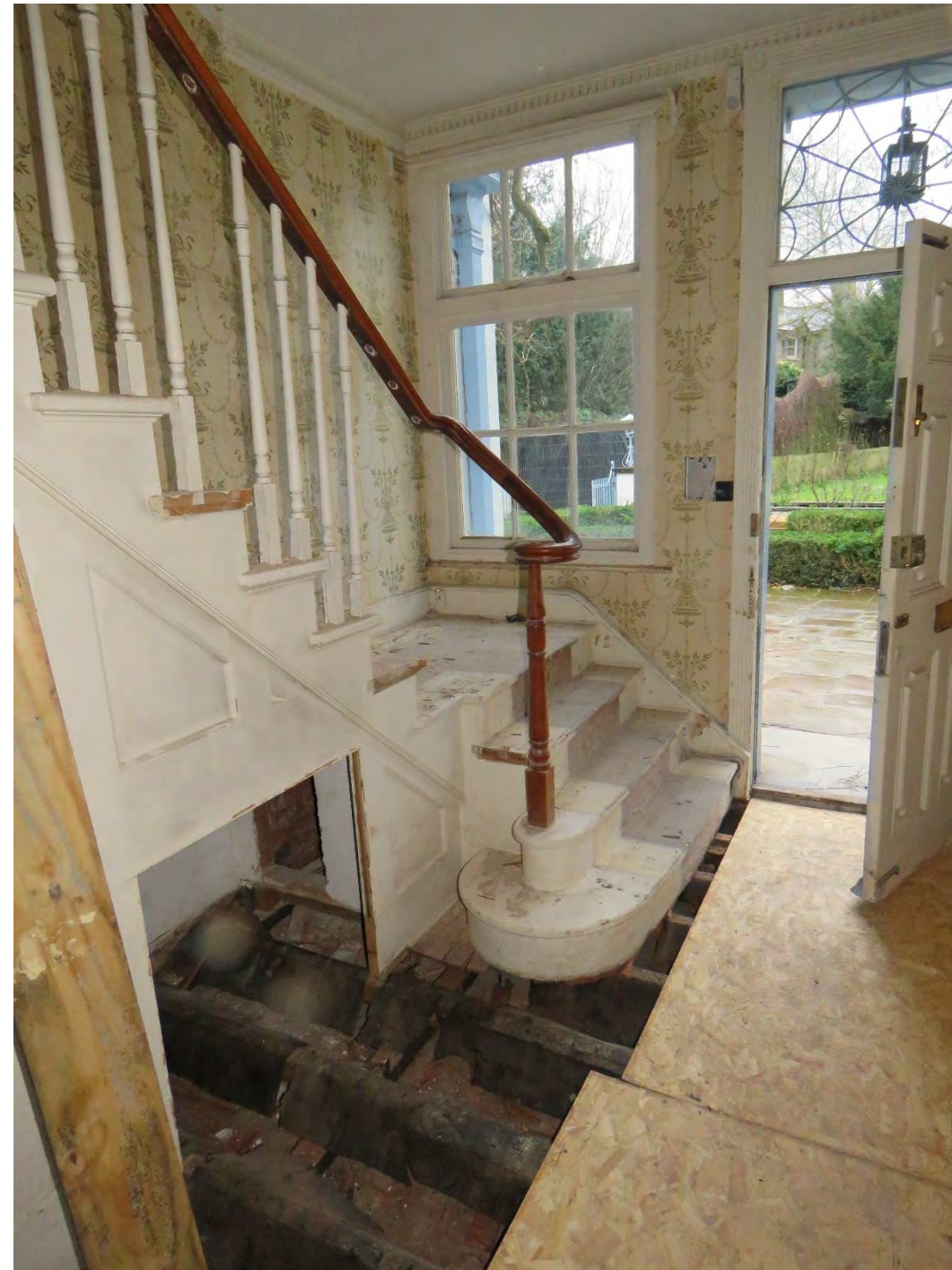
Figure 25: View of the entrance hall and staircase looking west. Though the staircase may visually be of an early-mid-20 th C date, its construction detailing appears modern ( Figure 26 ) and location is not original as the wall (with the window and entrance door) was brought forward during the c.1960s works. The insertion of the staircase in this location further necessitated blocking an opening from the Reception room ( Figure 24 )
