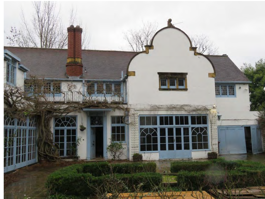
Figure 1: West Elevation of the main house. Note the original gable, chimney stacks and led windows (first floor)
