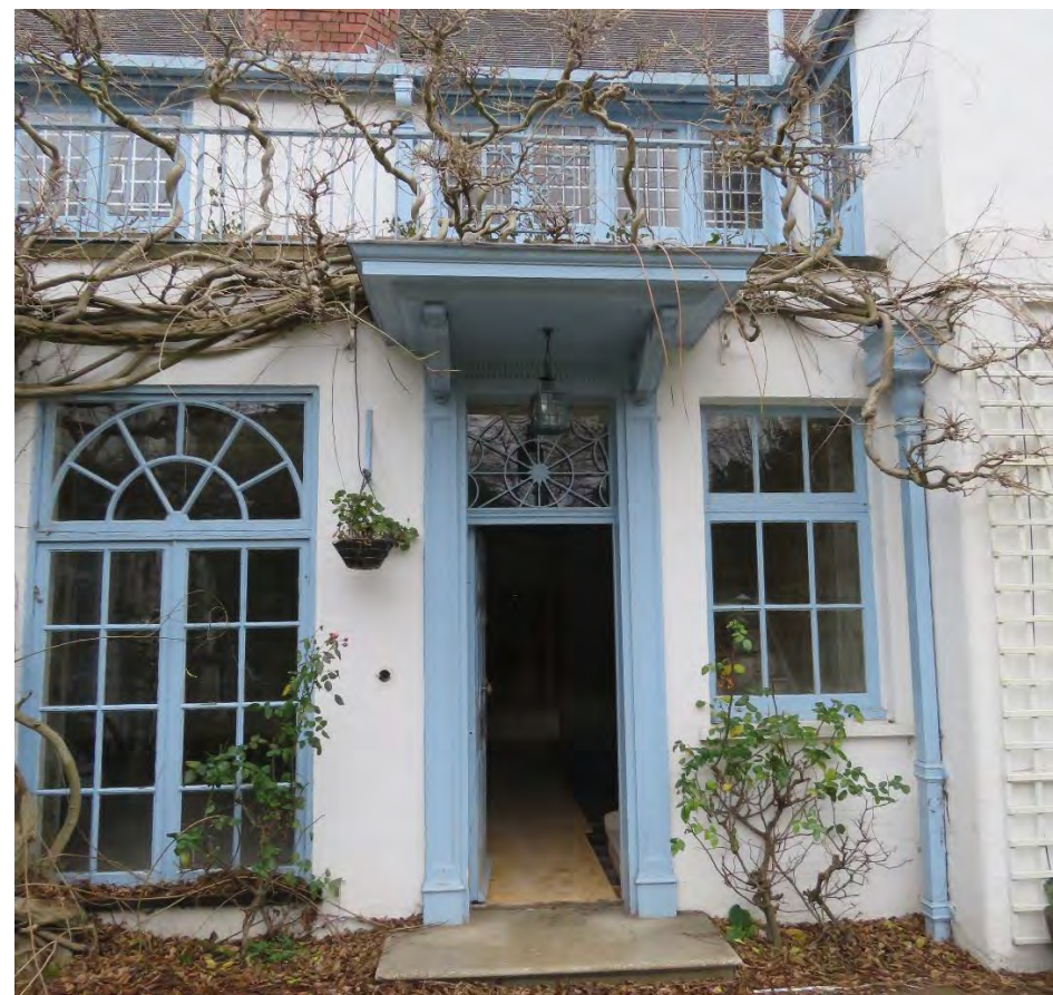
Figure 2: Detail of the front door and flanking fenestration. Note that the wall in this location was brought forward in the c.1960s. The door and windows are not original to the building.
