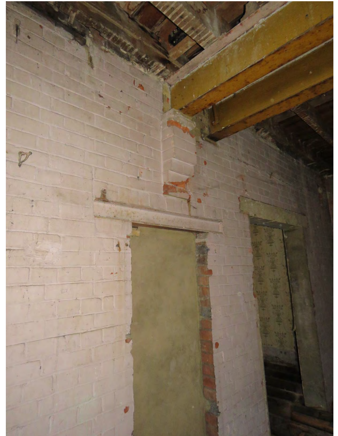
Figure 24: View of the two doorways leading to the Reception room from the entrance hall. The opening to the left (with a C channel lintel) is blocked, presumably when the staircase was added in its current location behind this. The second opening to the right has an RCC lintel and is modern.
