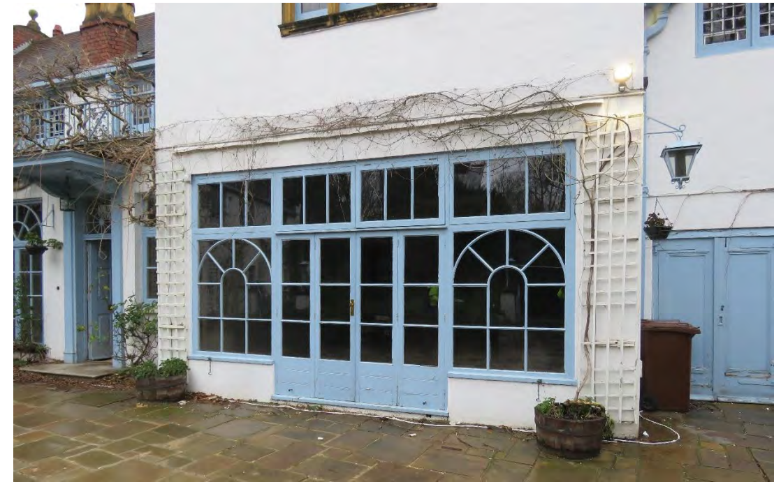
Figure 3: View of the conservatory style glazed French doors at the ground floor. This is a later intervention and replaced the original fenestration in this location during the c.1960s works.
