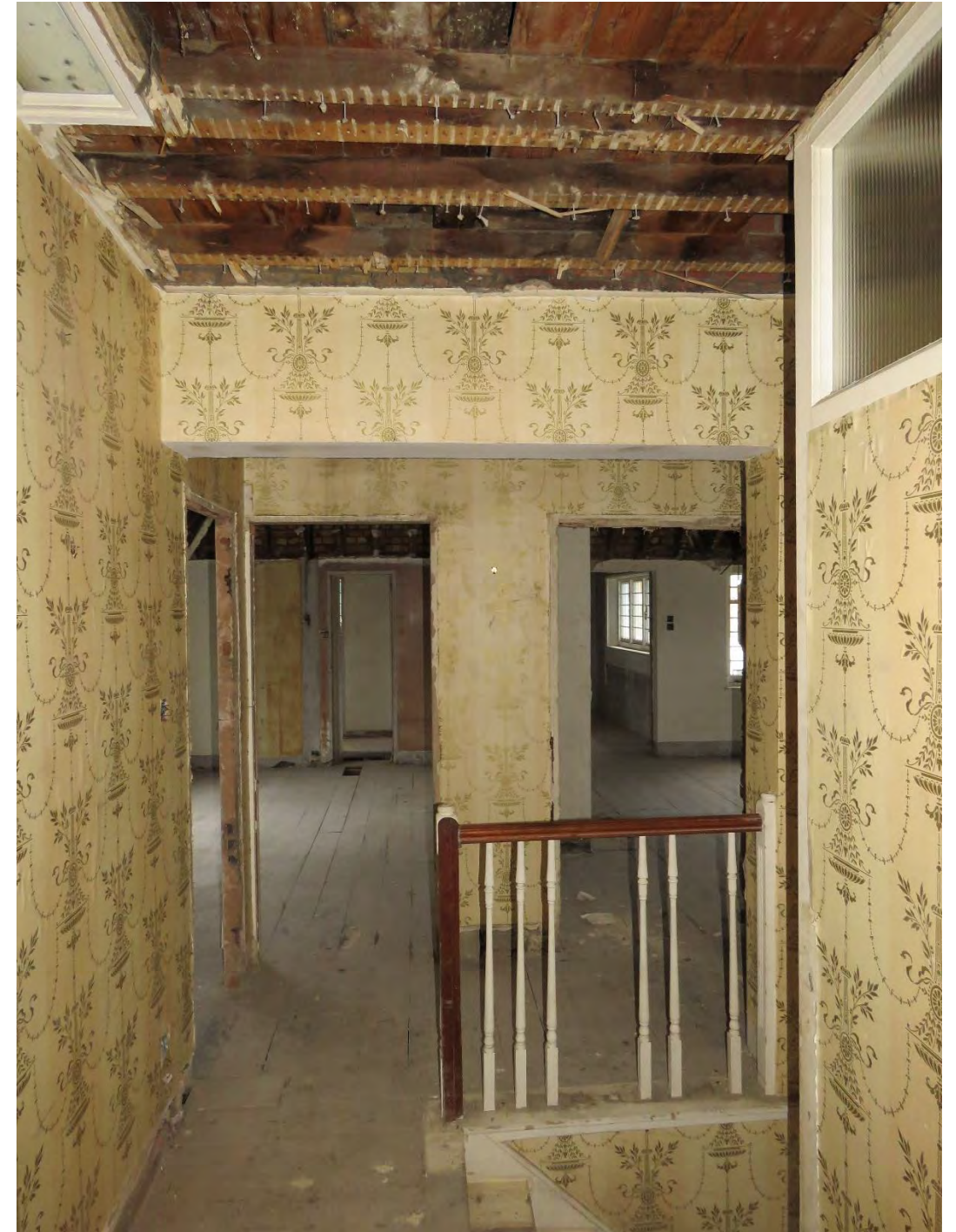
Figure 37: View of stair landing looking towards the south. The location of the original wall may be indicated by the downstand. The single brick and studwork partition with doorways leading to the bedrooms is modern. The floorboards in this area have been heavily altered.
