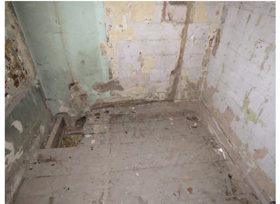
Figure 39: View of the rear wall of main building. Note the sporadic layers of construction within the walls and irregular floorboards. It appears this room has been heavily altered over time.
