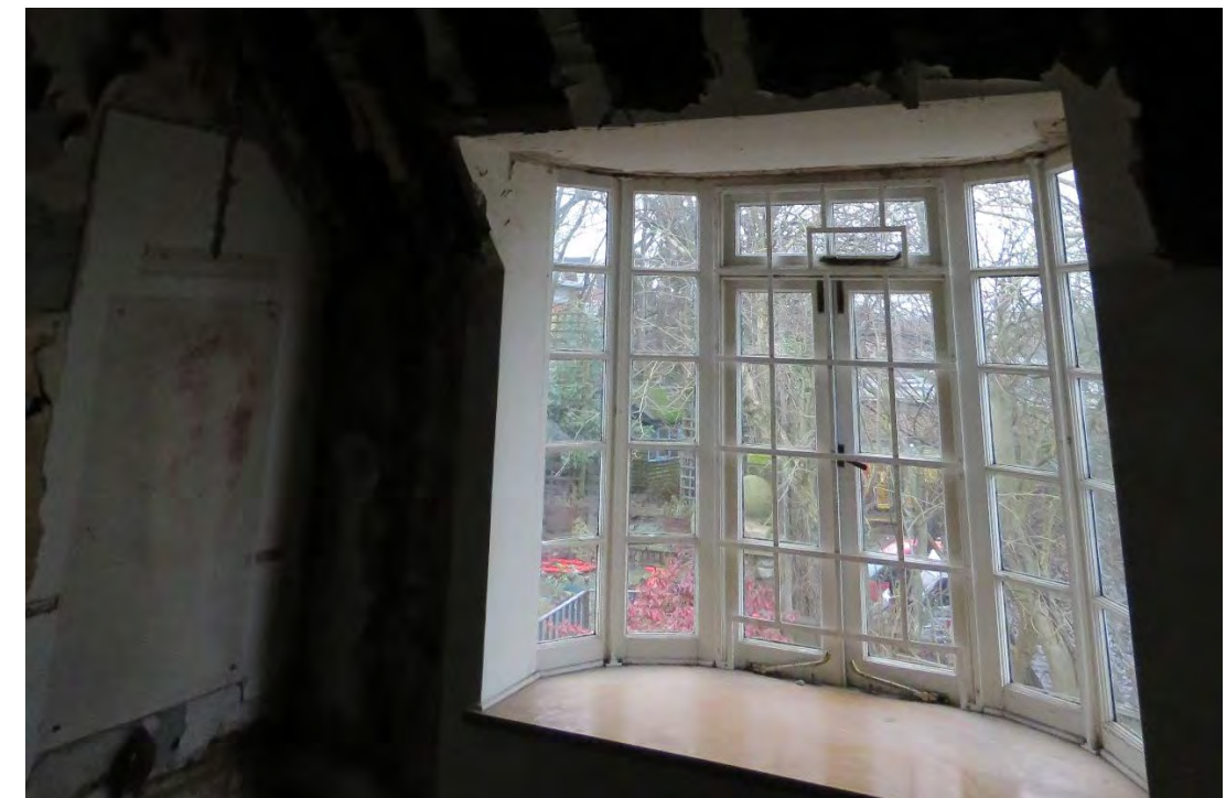
Figure 50: View of the c.1960s bay window. Note the chunky moulded sections, modern casement detailing and poorly proportioned glazing.
