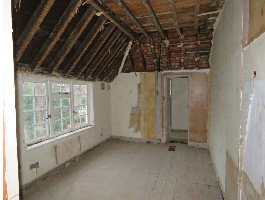
Figure 45: View looking south. Note the c.1960s windows on the east (rear) wall, modern narrow door openings and cement plastered walls. Floorboards in some areas are missing.
