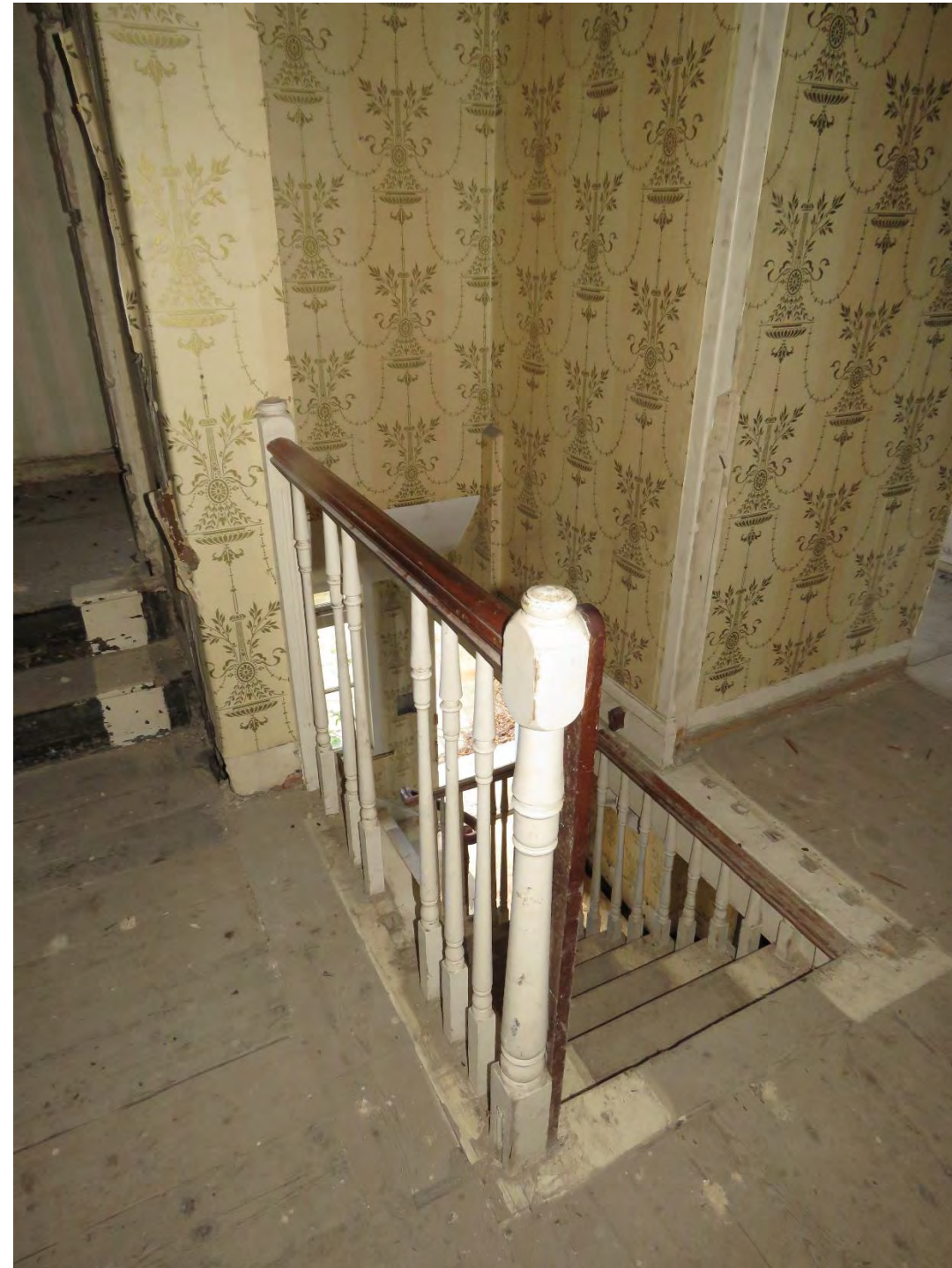
Figure 36: First floor staircase landing. This area has been heavily altered and the existing layout is not original.
