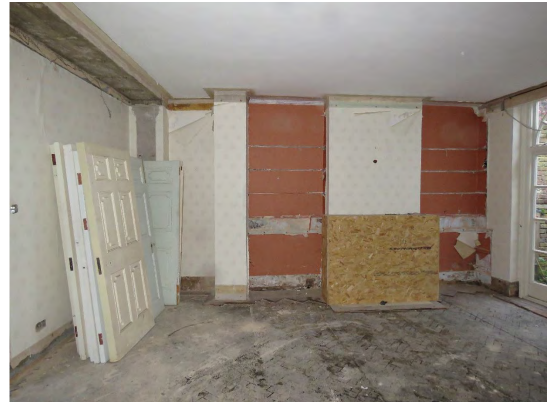
Figure 20: View of north wall showing the original chimney breast and the fireplace (protected in situ)
