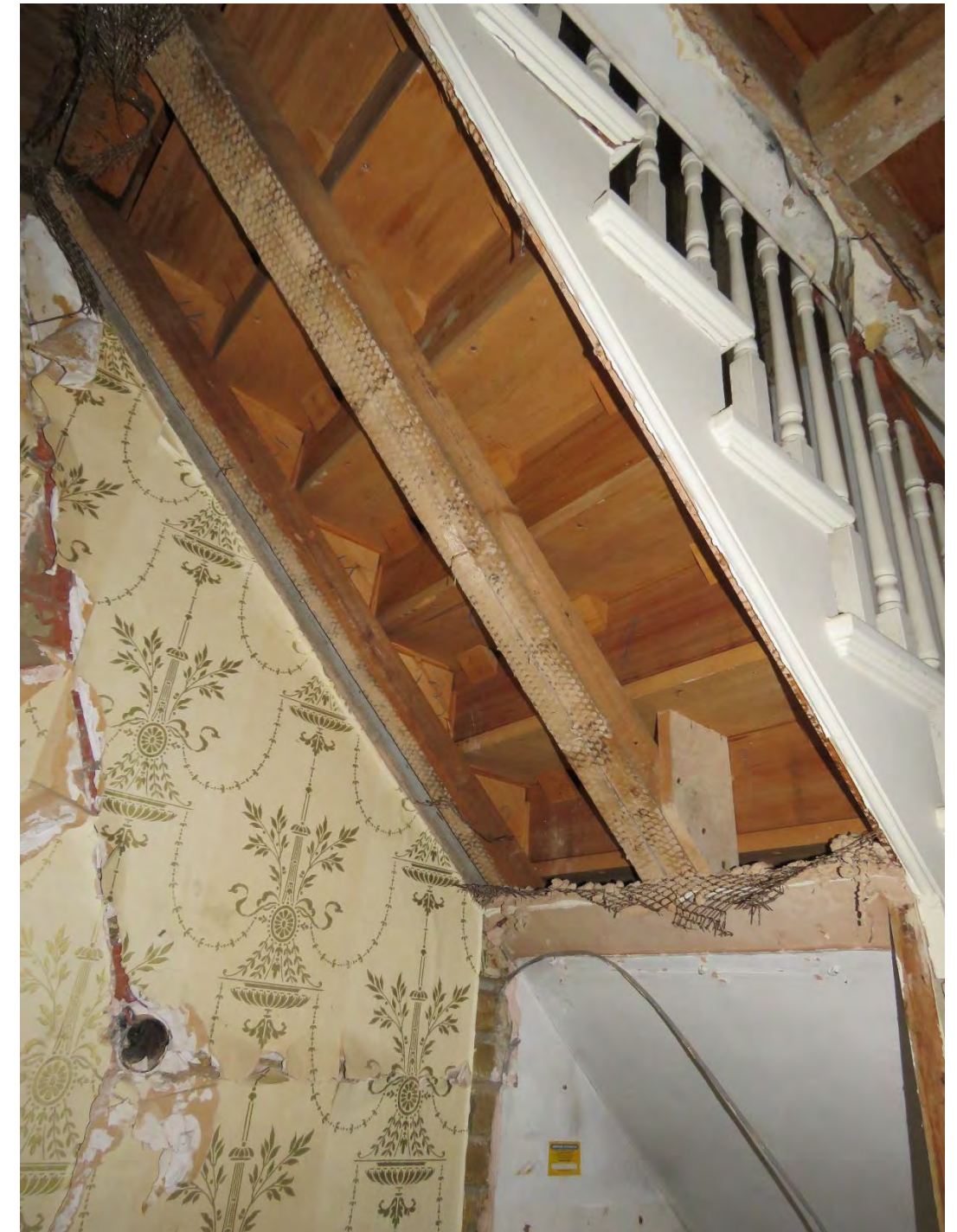
Figure 26: View of the underside of the staircase showing the modern stringer beam, treads and risers. The construction of the staircase appears to be modern.
