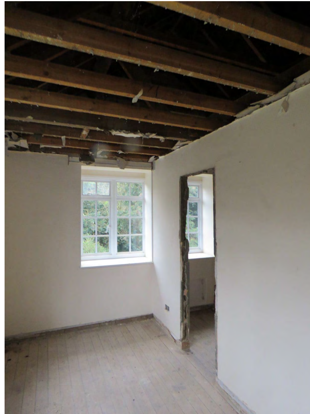
Figure 59: View of one of the rooms in the 1955-65 extension. Note the timber casement windows, modern studwork walls and cheap pine floorboards
