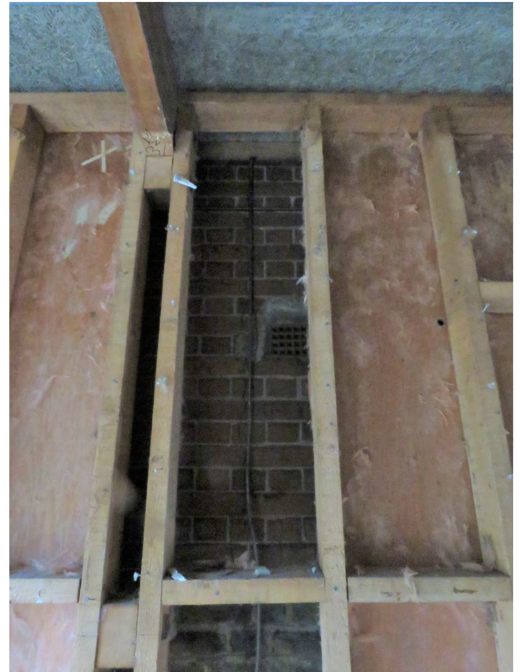
Figure 29: Detail of the timber studwork walls with plywood covering. Note the original exposed brick masonry behind. The house was originally brick faced and presumably transformed to its current 'whitewashed' form only after c.1969.
