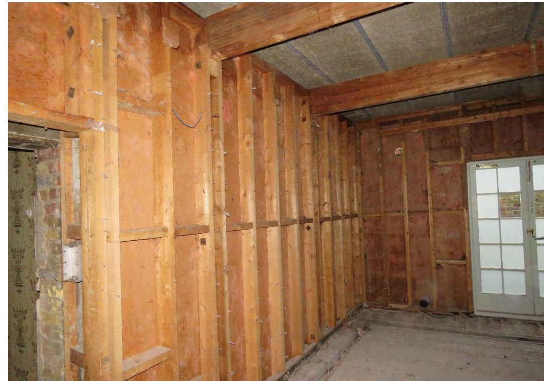
Figure 27: View of the c.1969 library extension. Note the timber studwork walls
