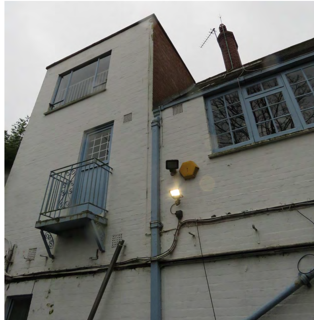
Figure 5: East elevation showing the garage extension to the left (south) with the additional (second storey). The window to the right appears to be a c.1960s addition.
