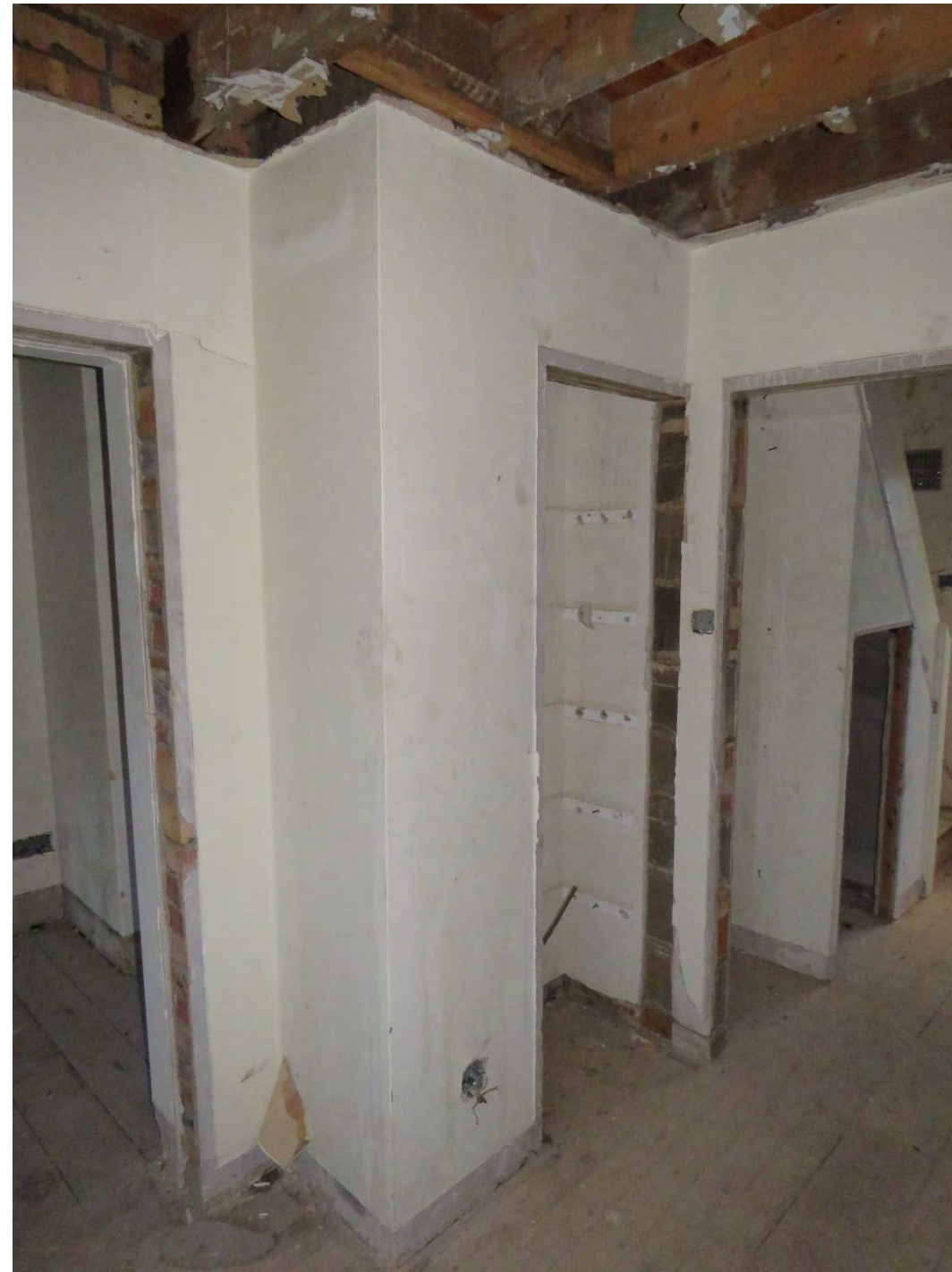
Figure 54: Modern studwork partitions in the dressing room area. The staircase leading to the second-floor bedroom is seen to the right.
