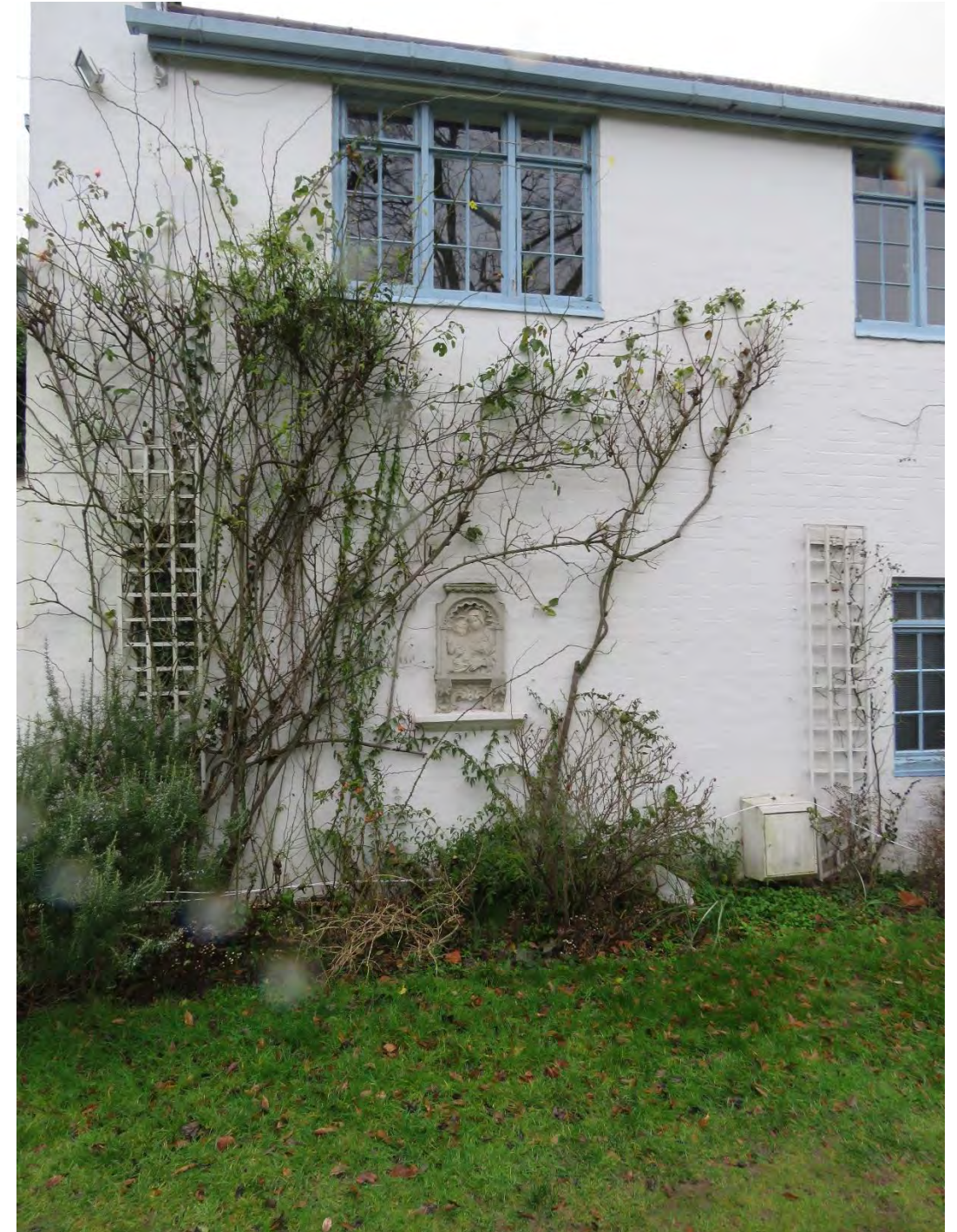
Figure 11: View of the south elevation of the 1955-65 wing. Note the timber casement windows.
