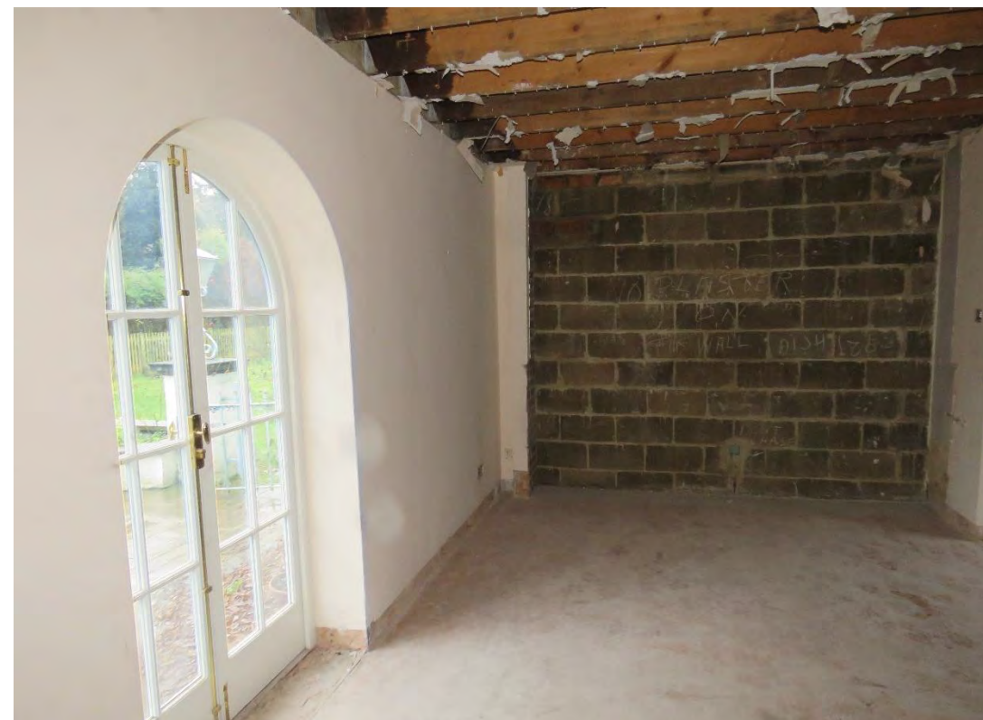
Figure 33: View of one of the rooms in the 1955-65 extension. Note the timber casement windows, modern studwork walls and cheap pine floorboards.
