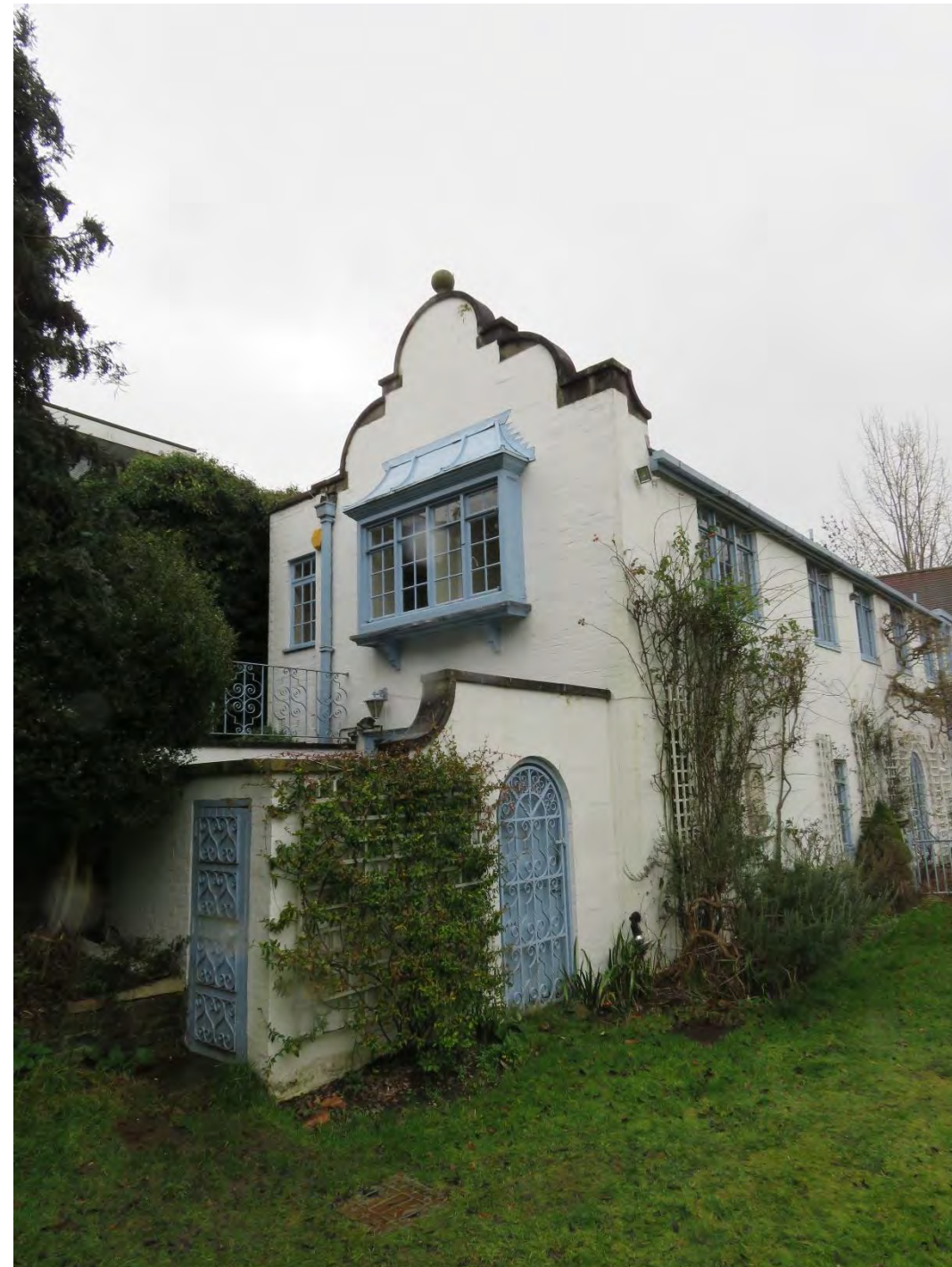
Figure 12: View of the west front of the 1955-65 wing. The gable 'apes' the original gable of the main house but the level of detailing is poor. The rectangular bay window with a small led roof is of poor-quality design. The projecting enclosure at ground floor further detracts from any meaningful reading of this elevation.
