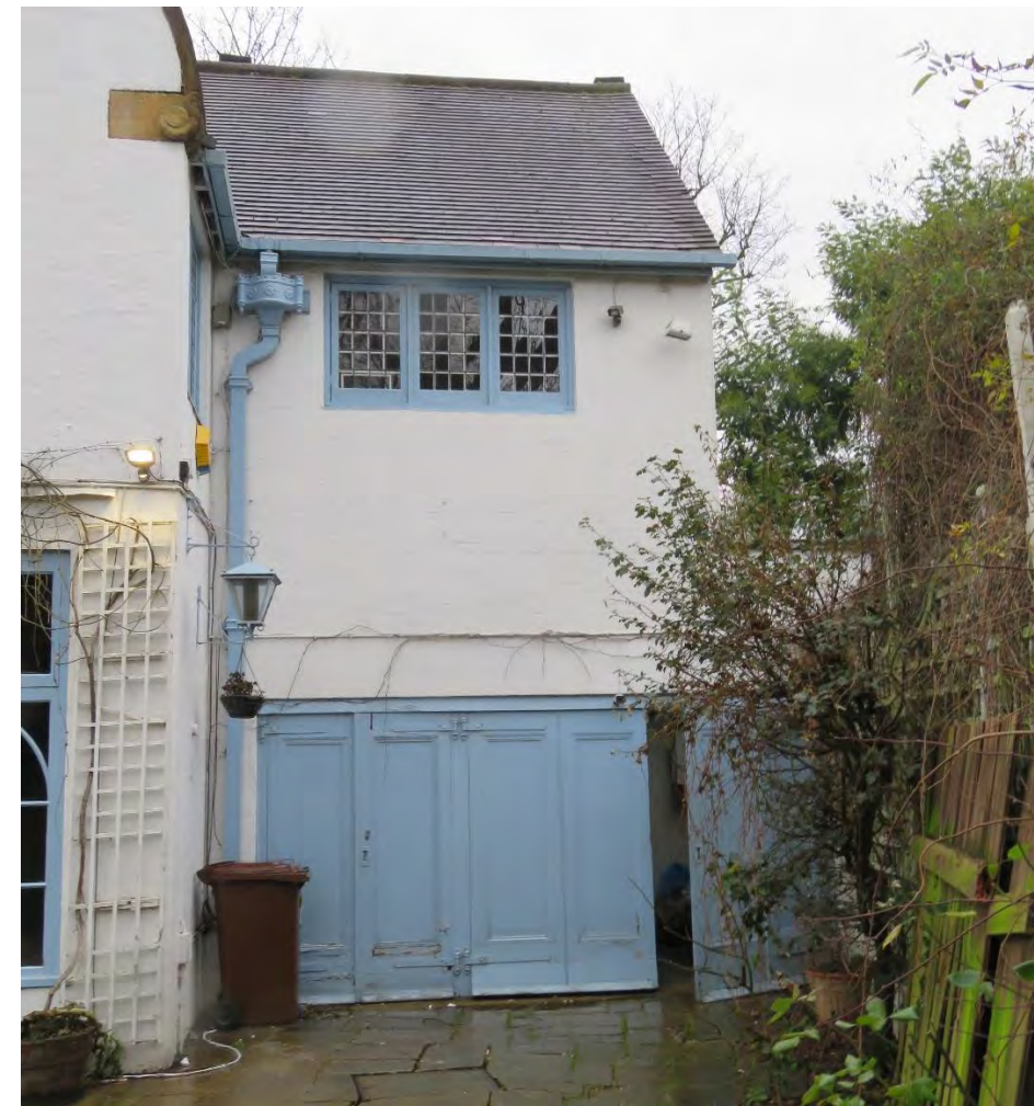
Figure 4: The garage extension to the south side of the house. This two-storey extension is not original to the building and was likely inserted in c.1960s.
