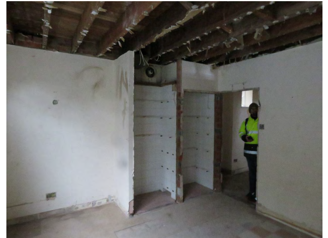
Figure 34: View of one of the rooms in the 1955-65 extension. Note the modern studwork partitions (forming the built-in furniture), half brick thick walls and linoleum flooring.
