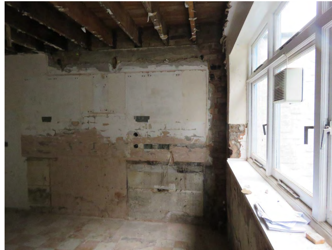
Figure 32: View of one of the rooms in the 1955-65 extension. Note the modern windows, cement plastered walls, linoleum floors and timber joist ceiling.
