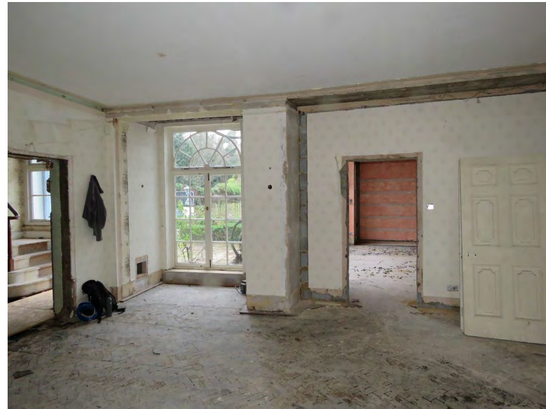
Figure 18: View of ground floor dining room. Note the original extent of the building line and the c.1960s extension with the French door (extended outwards)
