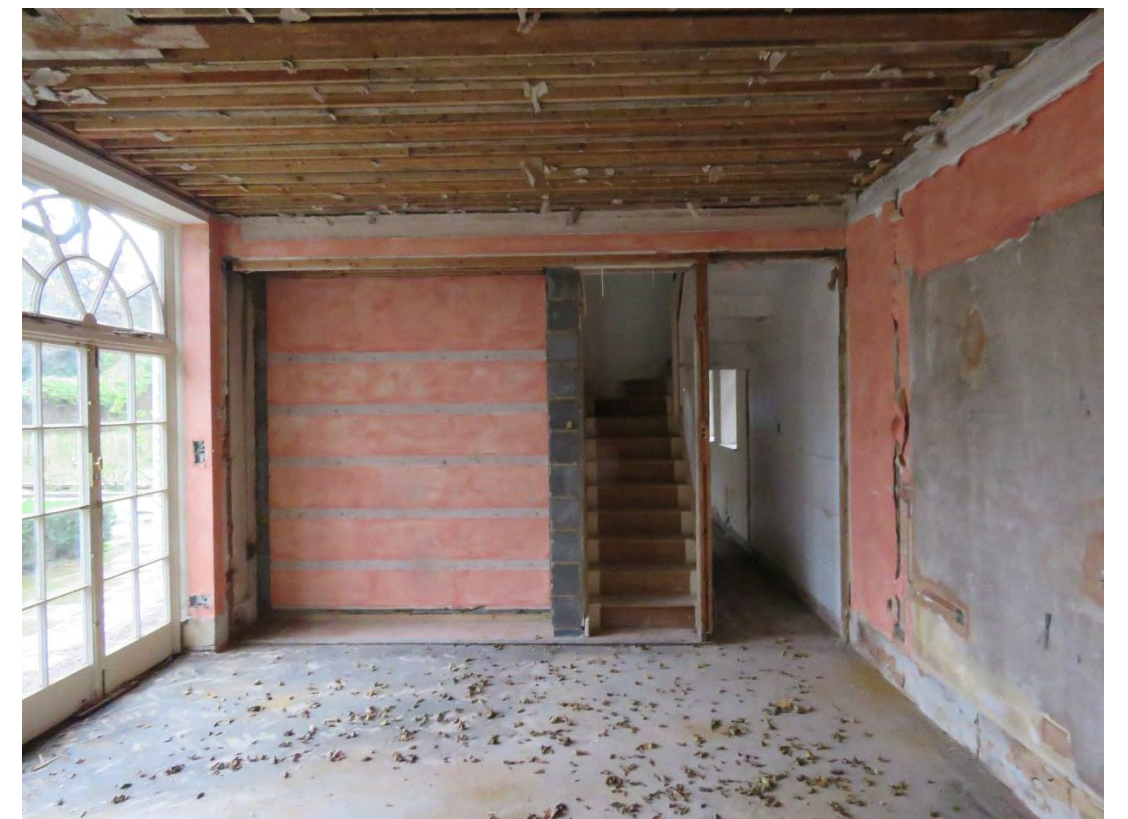
Figure 35: View of the 'Kitchen' area in the ground floor, part of the 1955-65 extension. Note the modern stairs, cement plastered walls and concrete screed floors.
