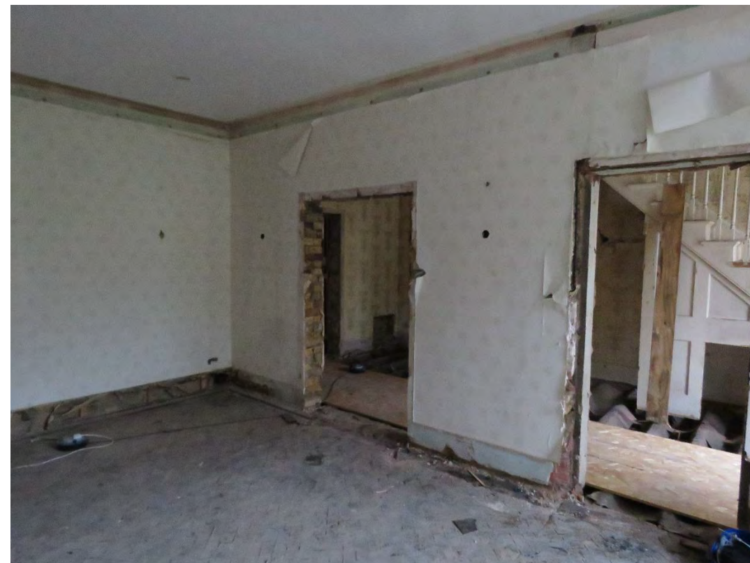
Figure 19: View of two doorways leading from the main entrance hall to the dining room. The door lintels are composed of channel sections, indicating that these were created at a later date.
