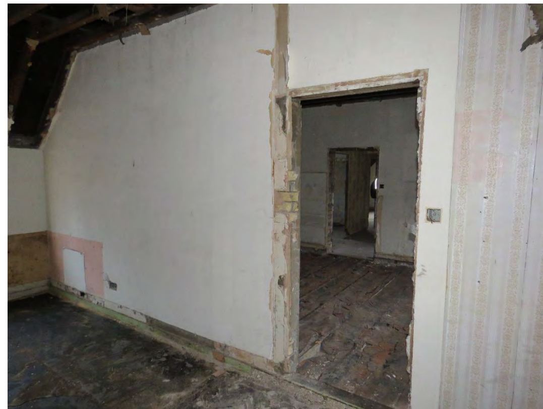
Figure 48: View looking southeast towards the Sitting room. Note the half brick thick modern partition wall dividing the rooms.
