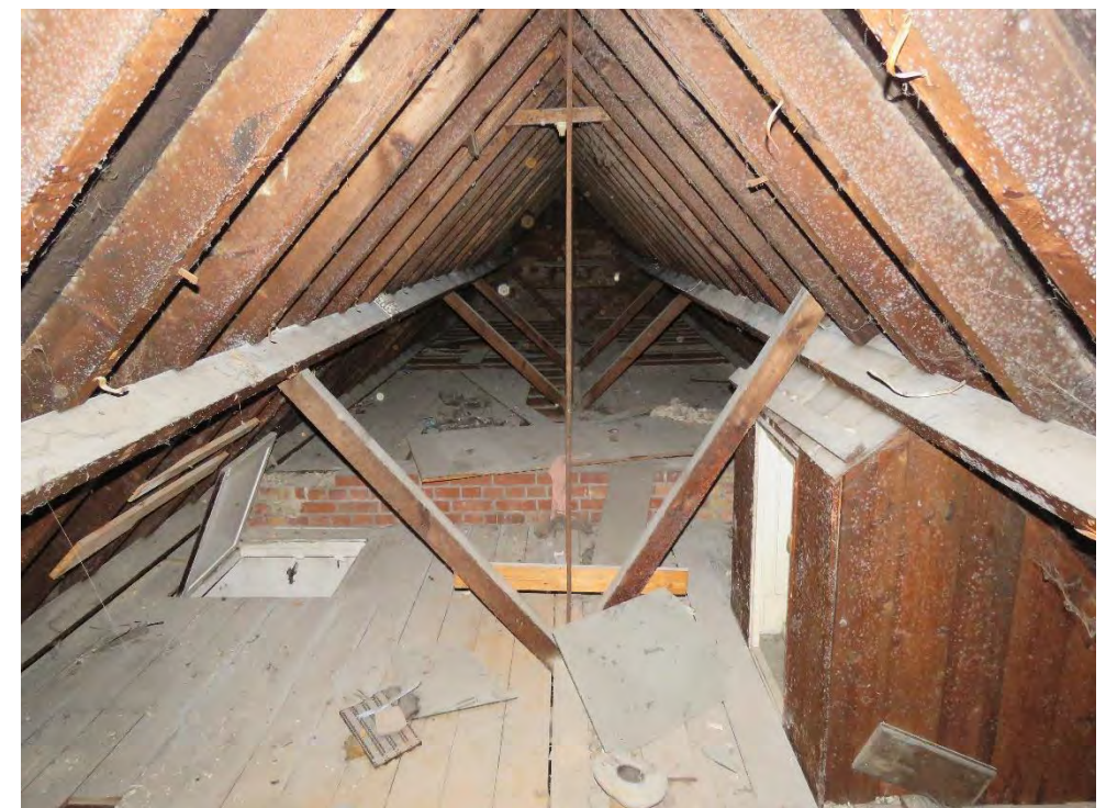
Figure 72: View of the cut roof construction through the main building and towards the north elevation.
