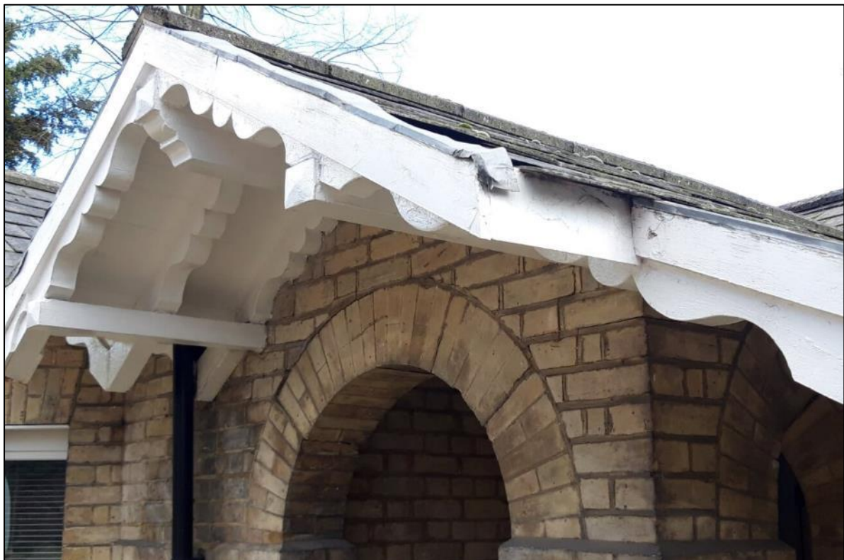
Photograph 9. A lifted tile presenting a crevice on the south-western elevation of the front porch gable.
