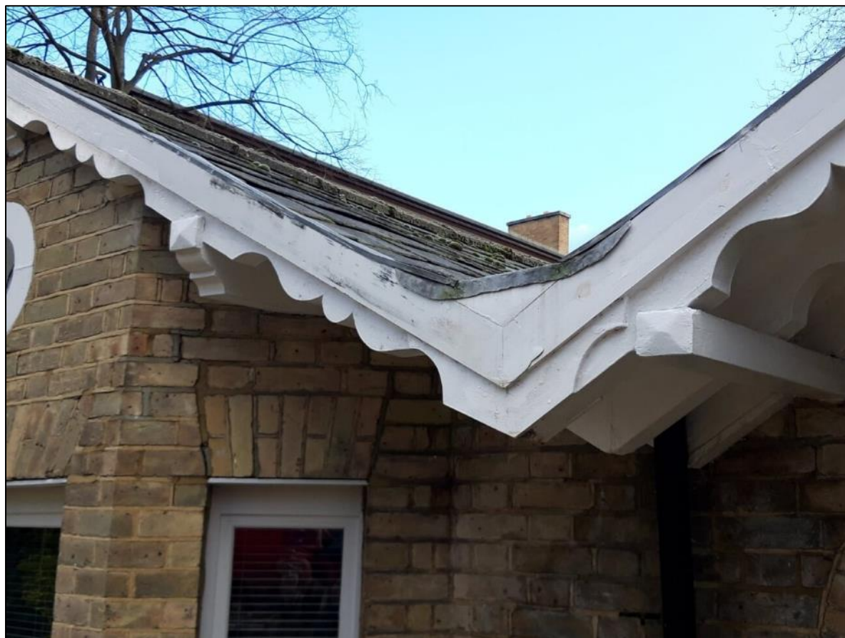
Photograph 10. A lifted tile in the valley between the front porch gable and north-west gable.
