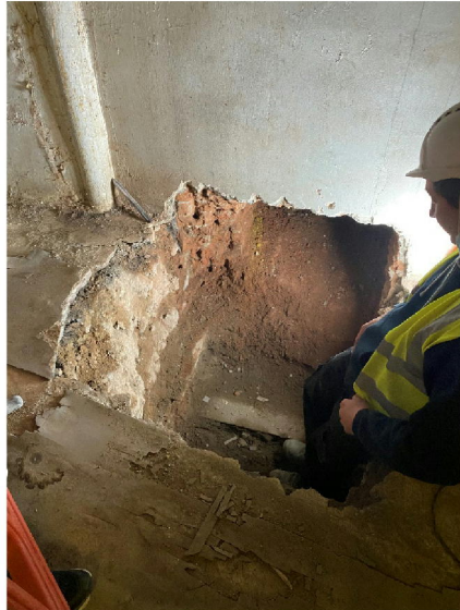
Photo 1 – Pit for underpin A dug out
