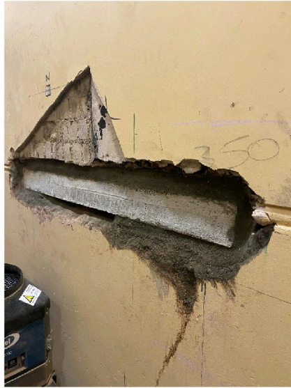
Photo 9 – Concrete lintel installed into wall to allow column starter installation
