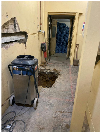
Photo 7 - Pit for underpin E being excavated Wall
