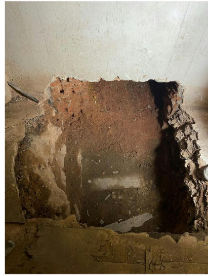
Photo 2 Pit for underpin A dug out
