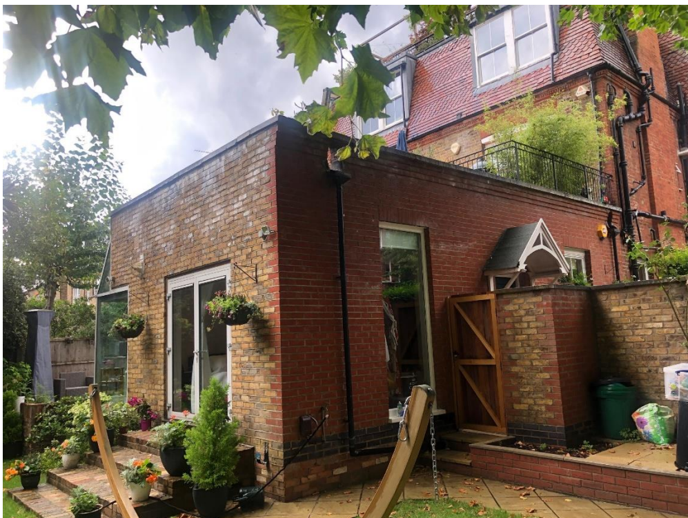
PHOTO 6 – Close up of extension side entrance from Fairhazel Gdns showing different bricks
