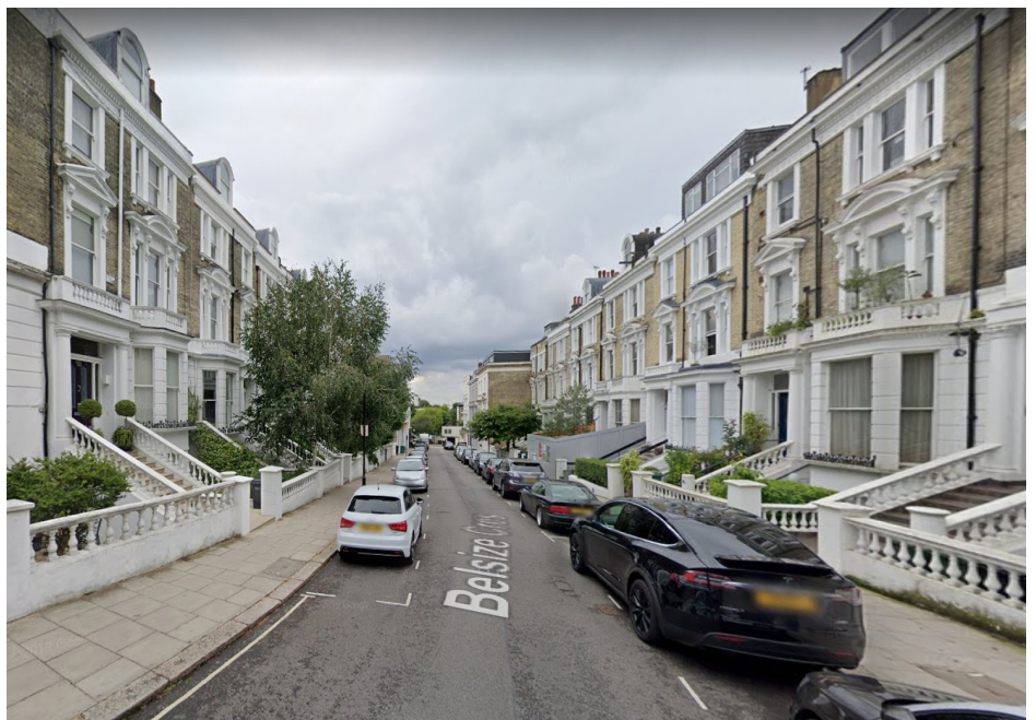
7 Belsize Crescent, front elevation. (general view from the top part of the Crescent).
