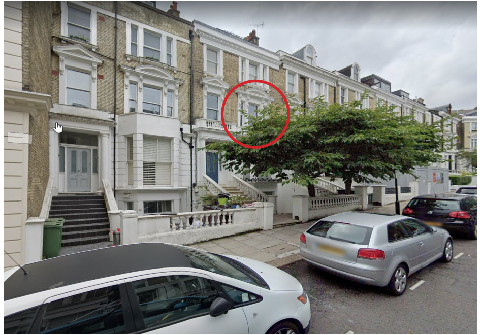
7 Belsize Crescent, front elevation. (view from the north side Belsize Village).
