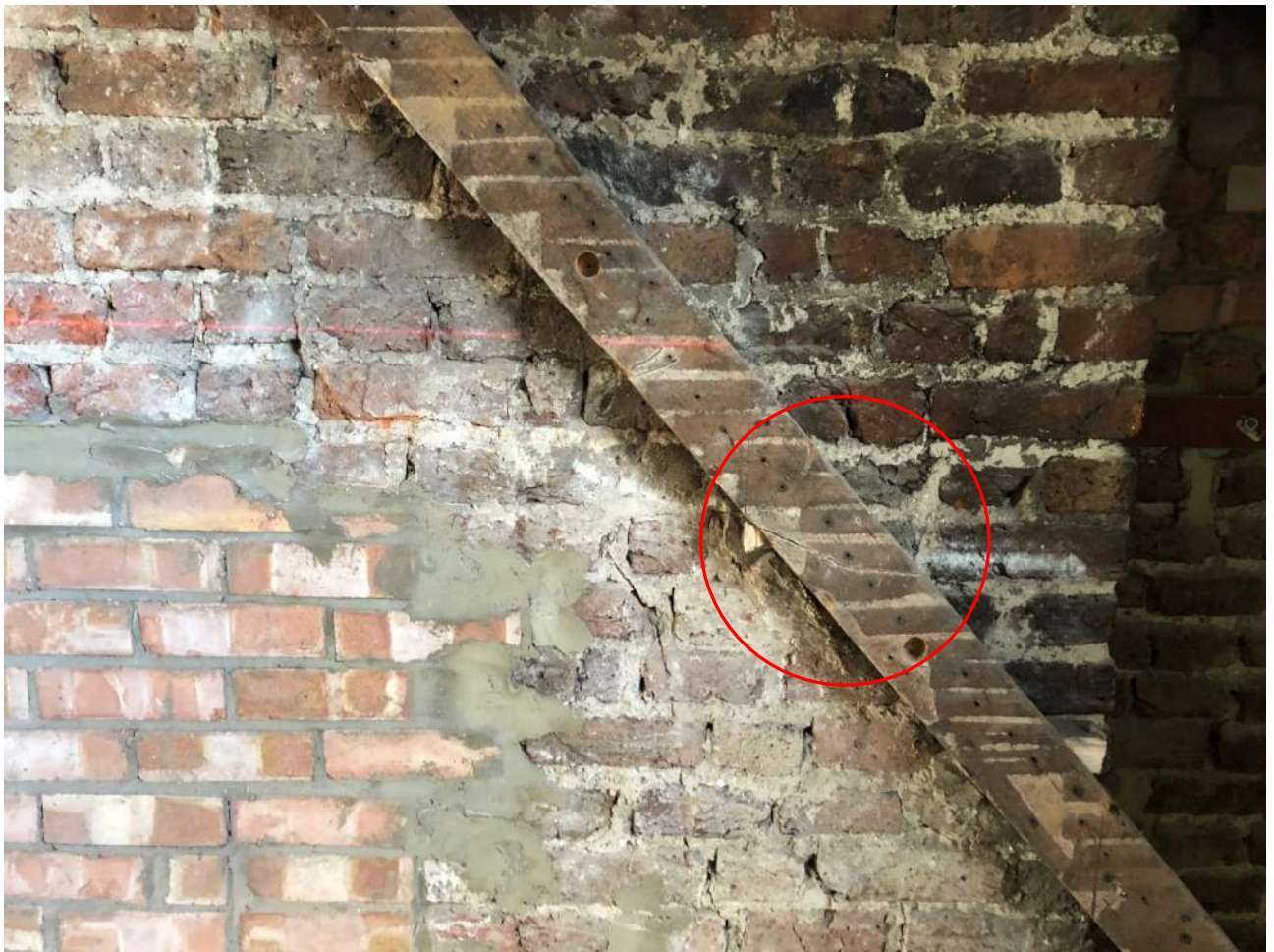
Fracture in diagonal brace
