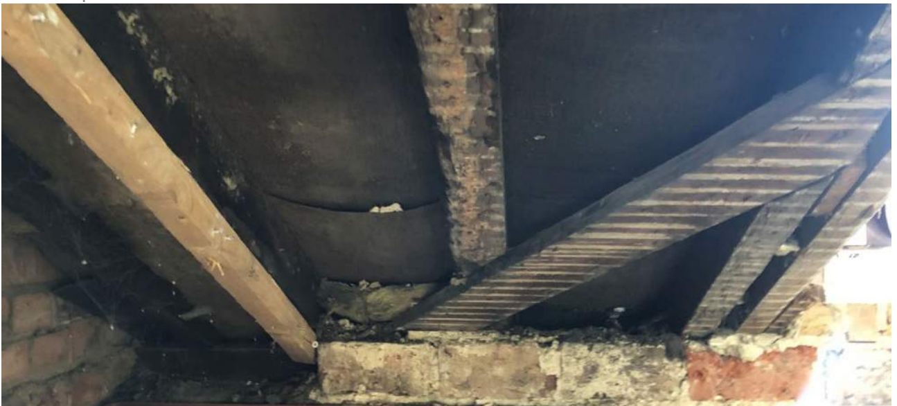
View of cut diagonal roof truss member.
