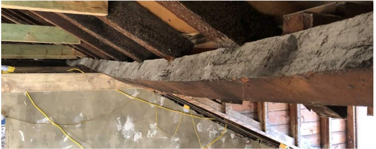
View along north purlin looking west showing continuity over spine wall and deflection at dormer heads.
