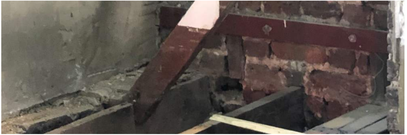
View of diagonal member of chimney breast frame work notched onto floor joist.
