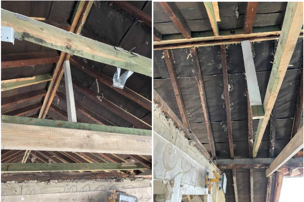
View of new ridge beams and central strut/truss.
