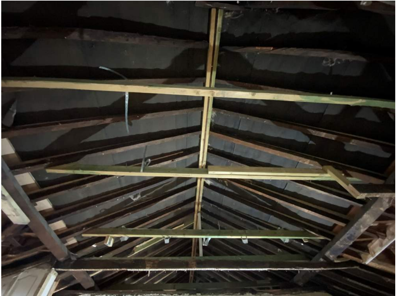
View of modern tie beams across the roof and firring pieces on top of the rafters
