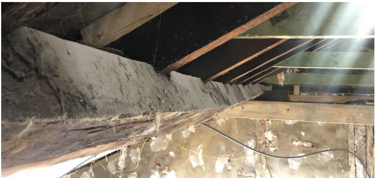
View along south purlin looking west again showing continuity and deflection.
