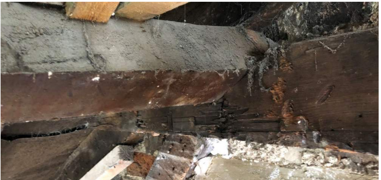
View of purlin notched into chimney breast beam.
