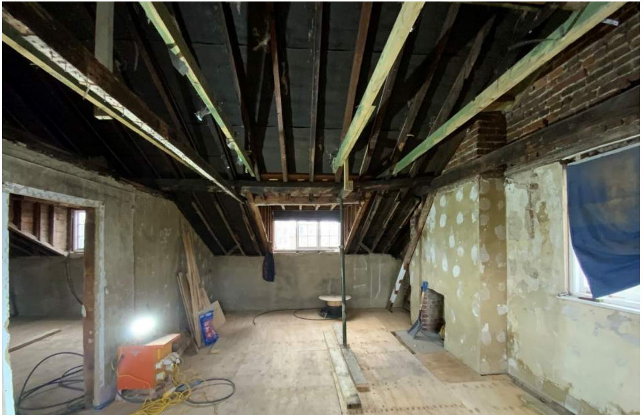
General view of the roof space looking south on the western side of the house, showing fractured purlin and modern timber roof elements.
