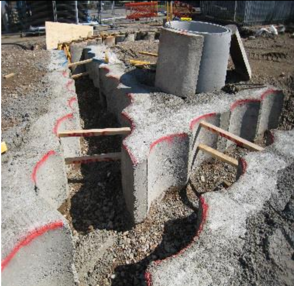
Figure 4 - Guide wall constructed
