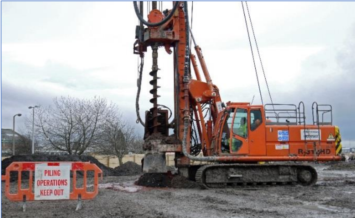
Figure 5 - CFA Pile rig
