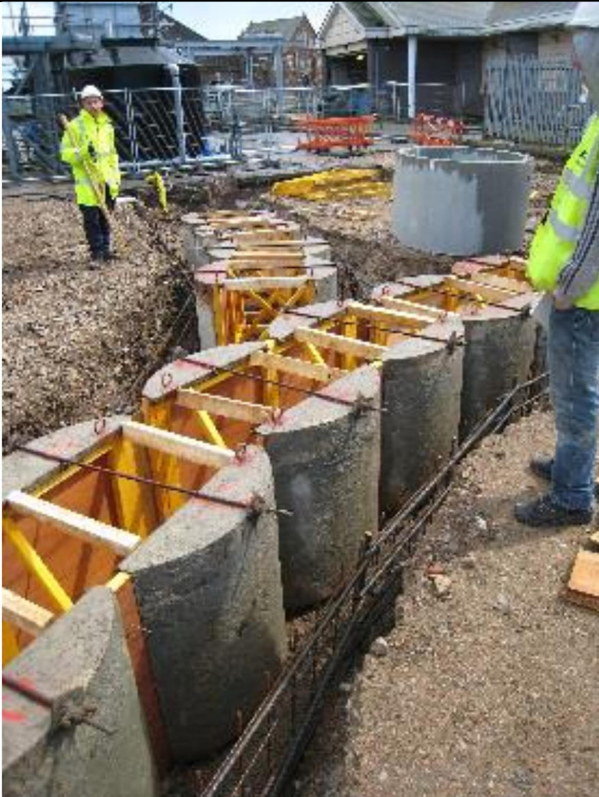
Figure 3 - Guide wall scallop formwork
