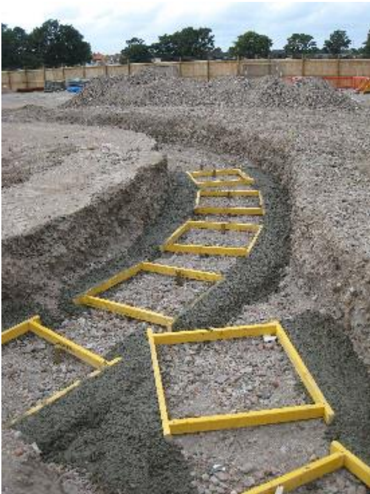
Figure 2 - Guide wall formation
