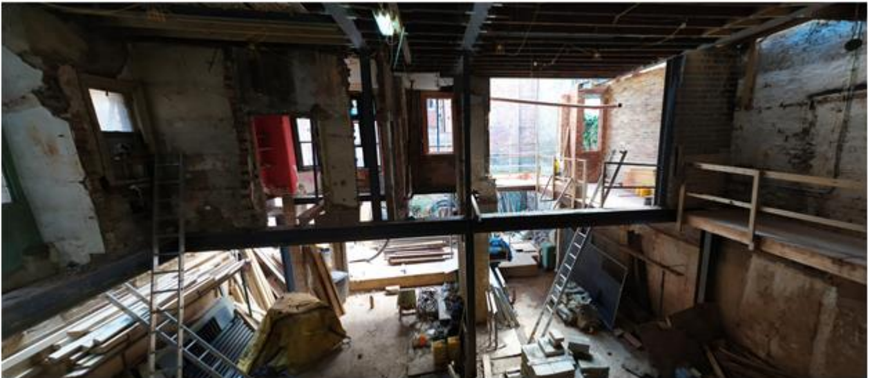
Figure 19: View of excavated basement which extends to rear boundary
