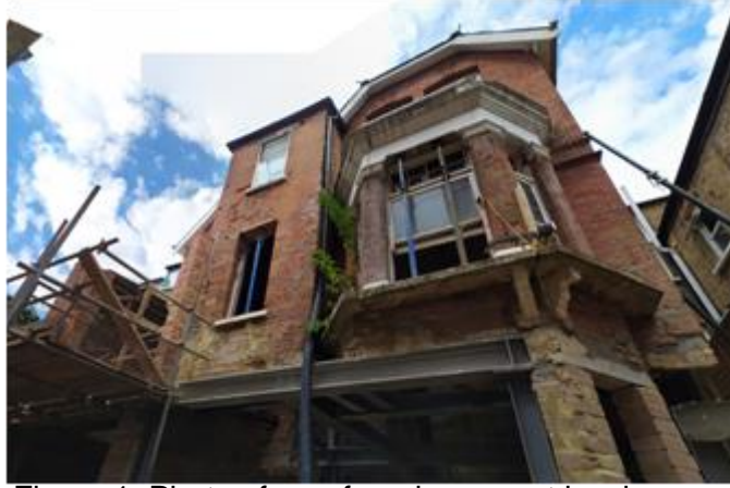
Figure 1: Photo of rear from basement level
