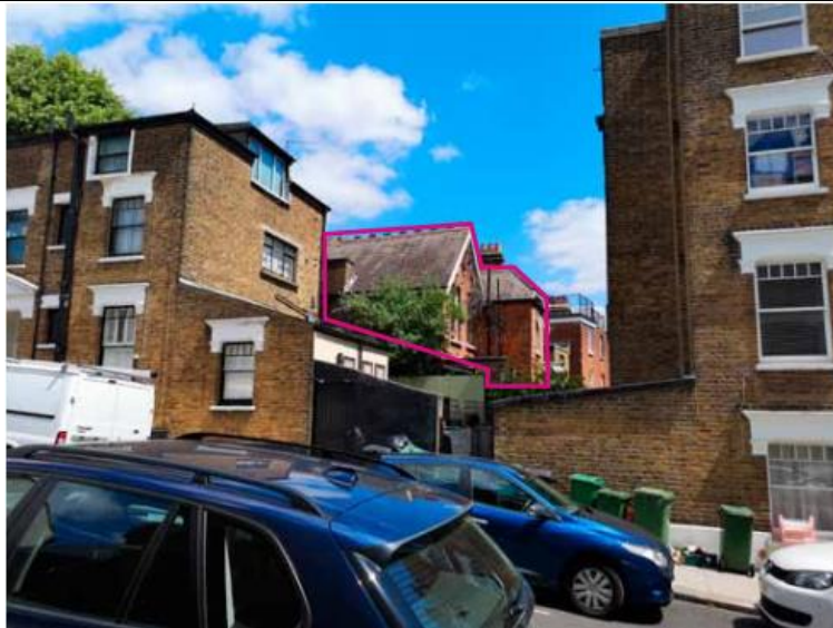
Figure 12: View of rear from Gondar Gardens
