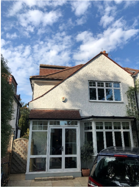
Photos of Existing Building- Front
