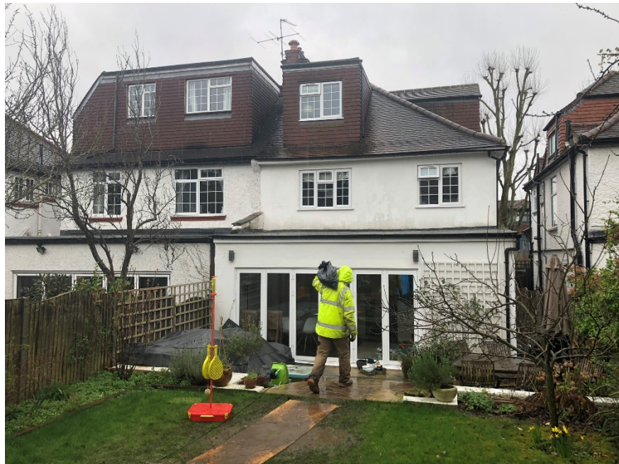
Photos of Existing Building- Rear
