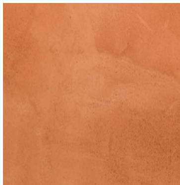
CEILING AND WALL: RED LIME FINISH 104
