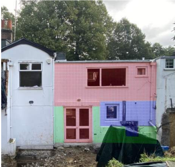
Central range rear façade with modern fabric highlighted in red. Assumed modern fabric is highlighted in blue and assumed historic fabric highlighted in green
