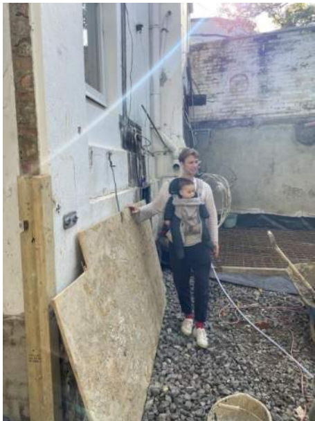
Photograph showing the steps in the rear façade
