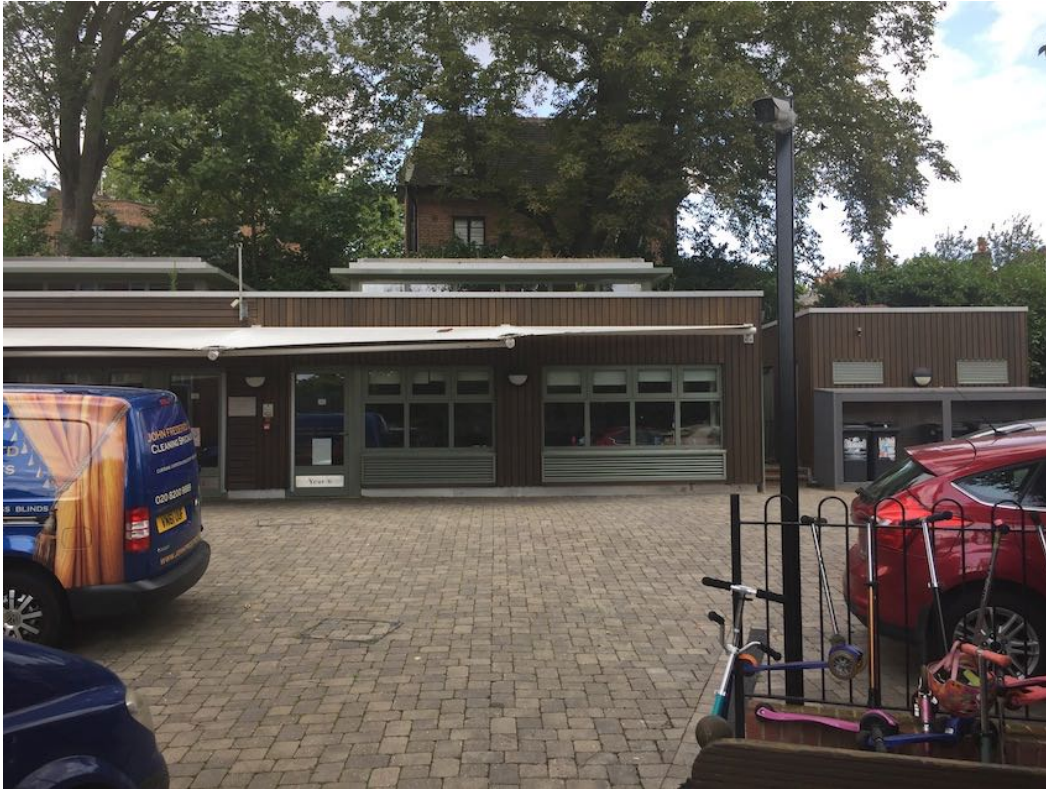
View of the eastern classroom, with plant room to the right, and car park area in front
