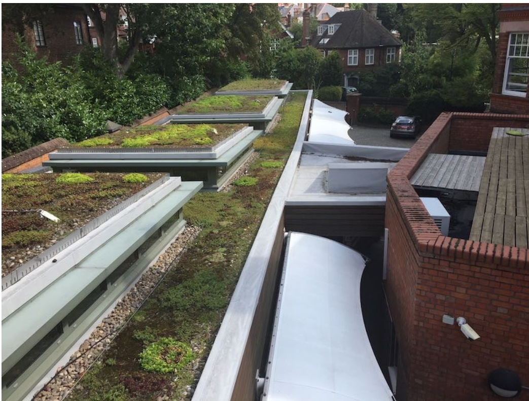
View of the roofs of the Classroom block, with raised lanterns and green sedum roof planting, and the canvas awning canopies to the right side
