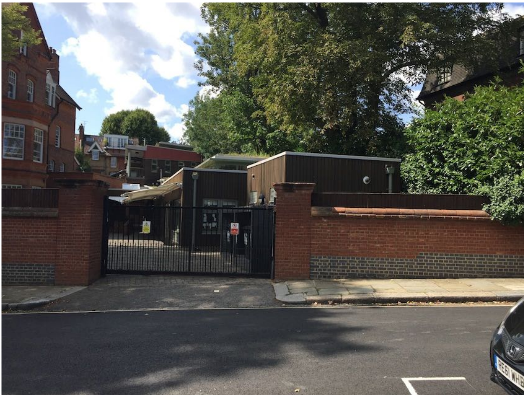
View of north Classrooms block from Belsize Lane, at the vehicular entrance to the site
