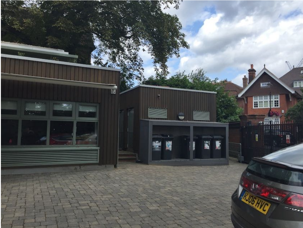
View of the eastern classroom, with plant room to the right, and car park area in front
