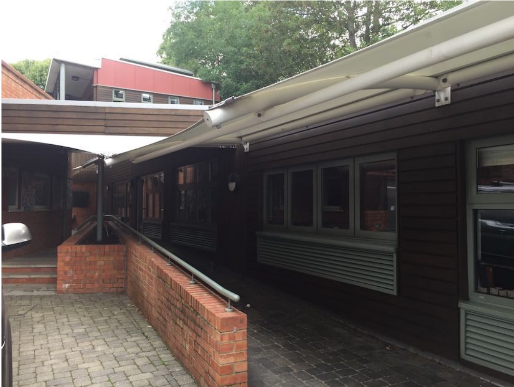
View of the "link" area with external covered space at steps and ramp
