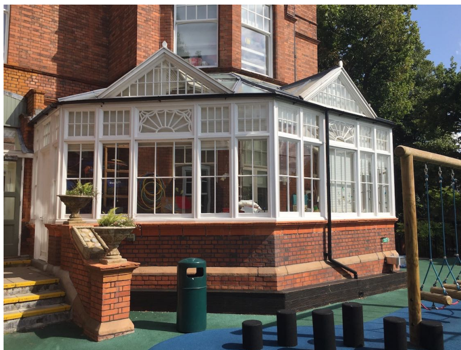
Photo of the original “Orangery” on the south side of the main house
