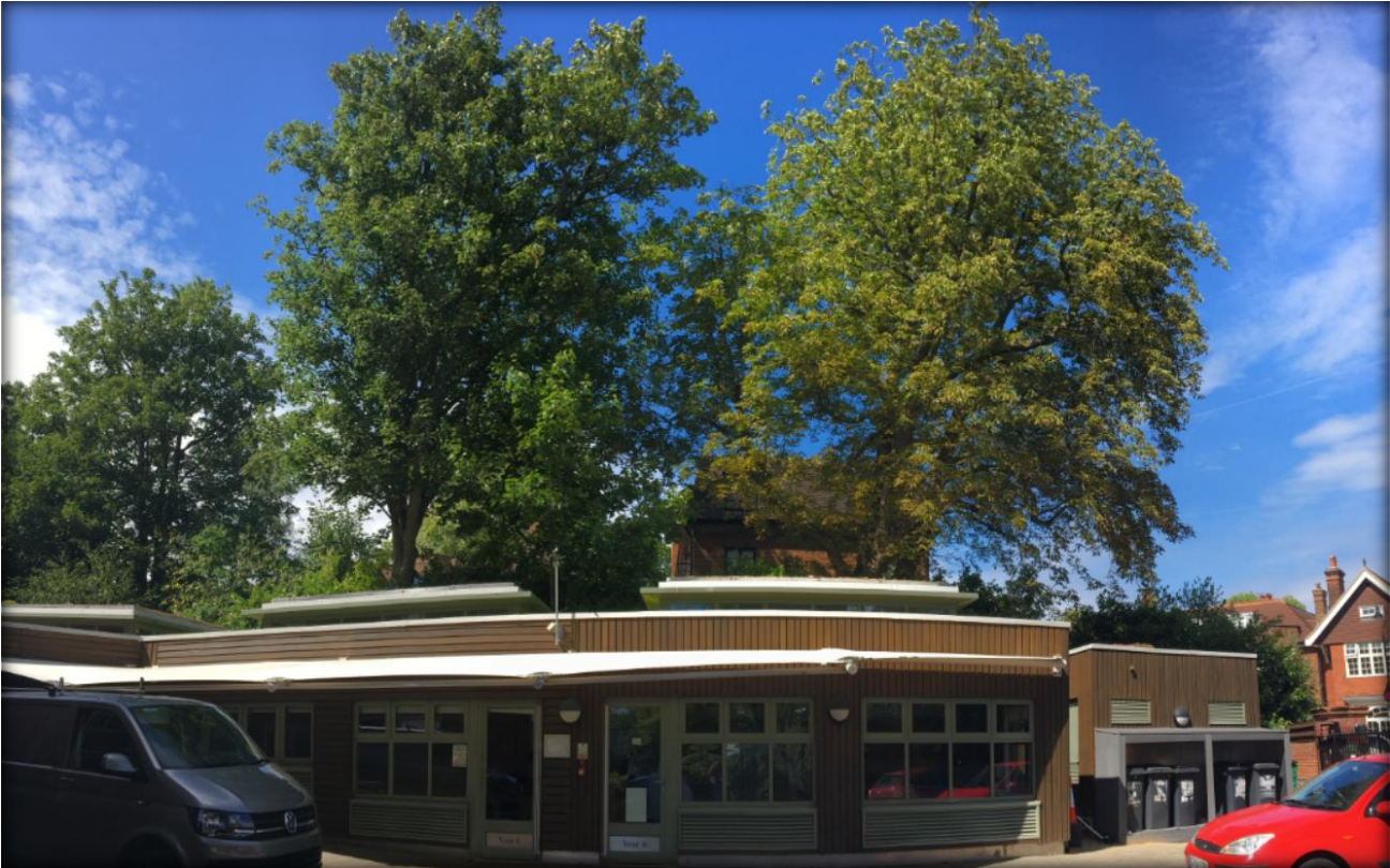
Figure 2: Photograph Showing the Site as Viewed from the South.
