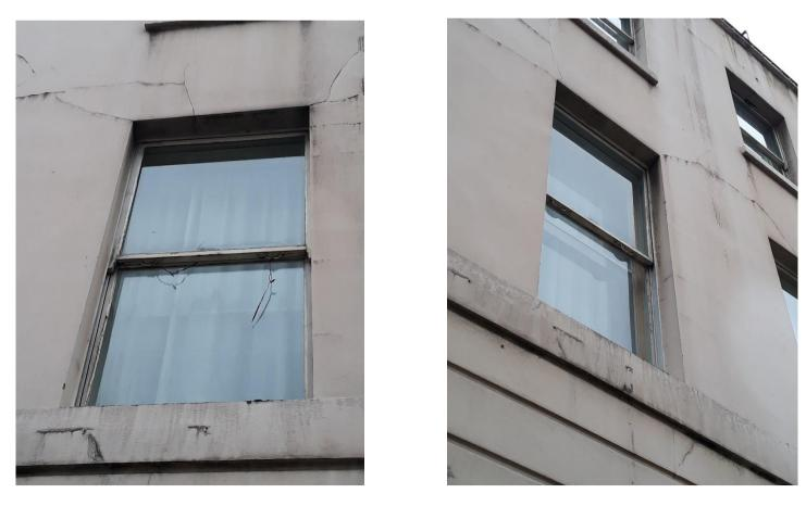
Cut out render 50mm each side of crack and make good with new sand and cement render 6 parts sand, 1 part cement, 1 part lime
