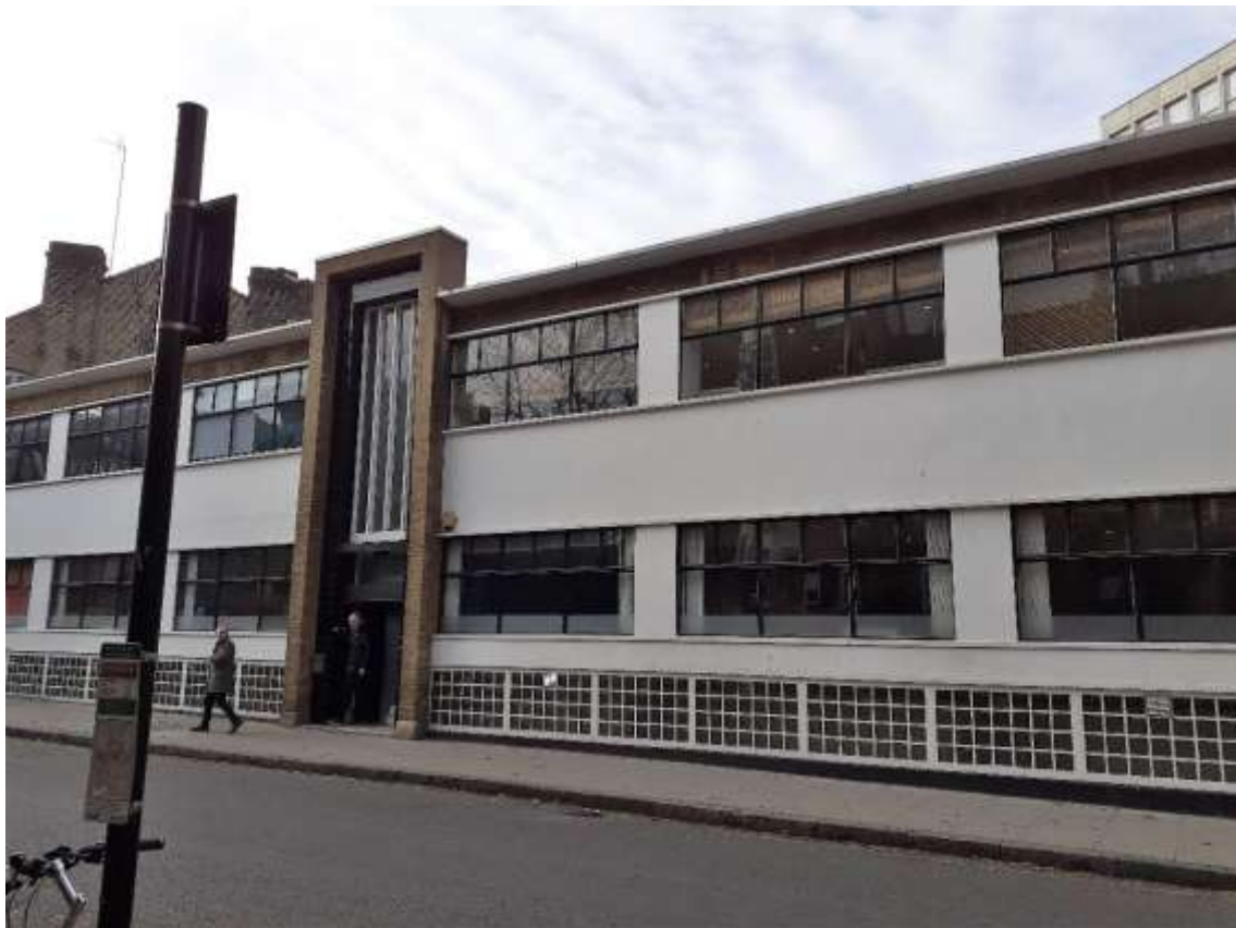
Image 1: 20 Flaxman Terrace, 1950s Extension – Illustrating the existing solid opaque glass blocks on the facade
