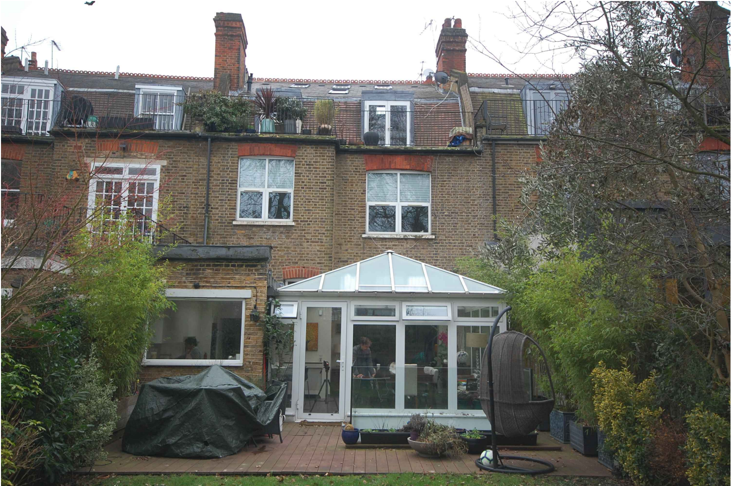
EXISTING REAR ELEVATION OF HOUSE
