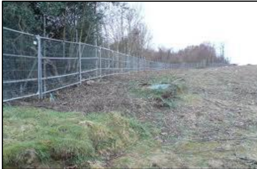
Tree protective fencing example.
