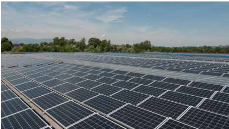
Slovenia Installation: 150 kW | S-Dome System
