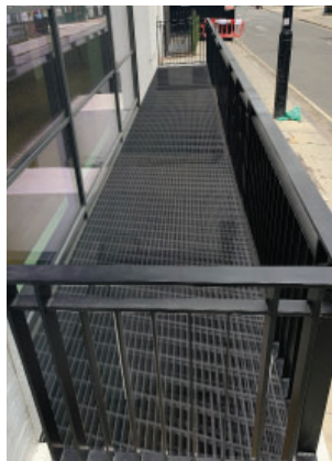
PROPOSED GRATING PANELS TO LIGHTWELL
