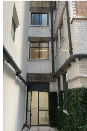
EXISTING WINDOW IN INTERNAL PATIO/ LIGHTWELL
