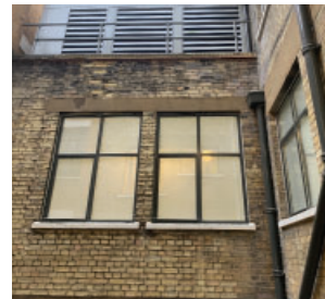
EXISTING WINDOW IN INTERNAL PATIO/ LIGHTWELL
