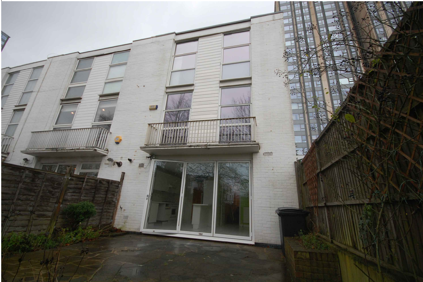
rear elevation facing south
