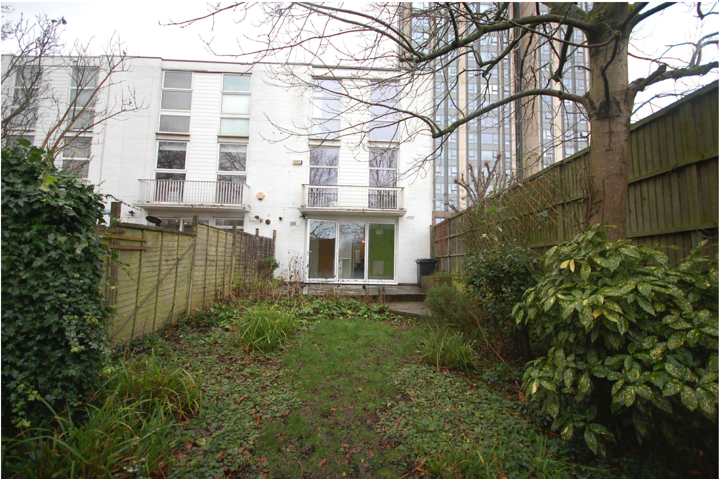
rear elevation facing south
