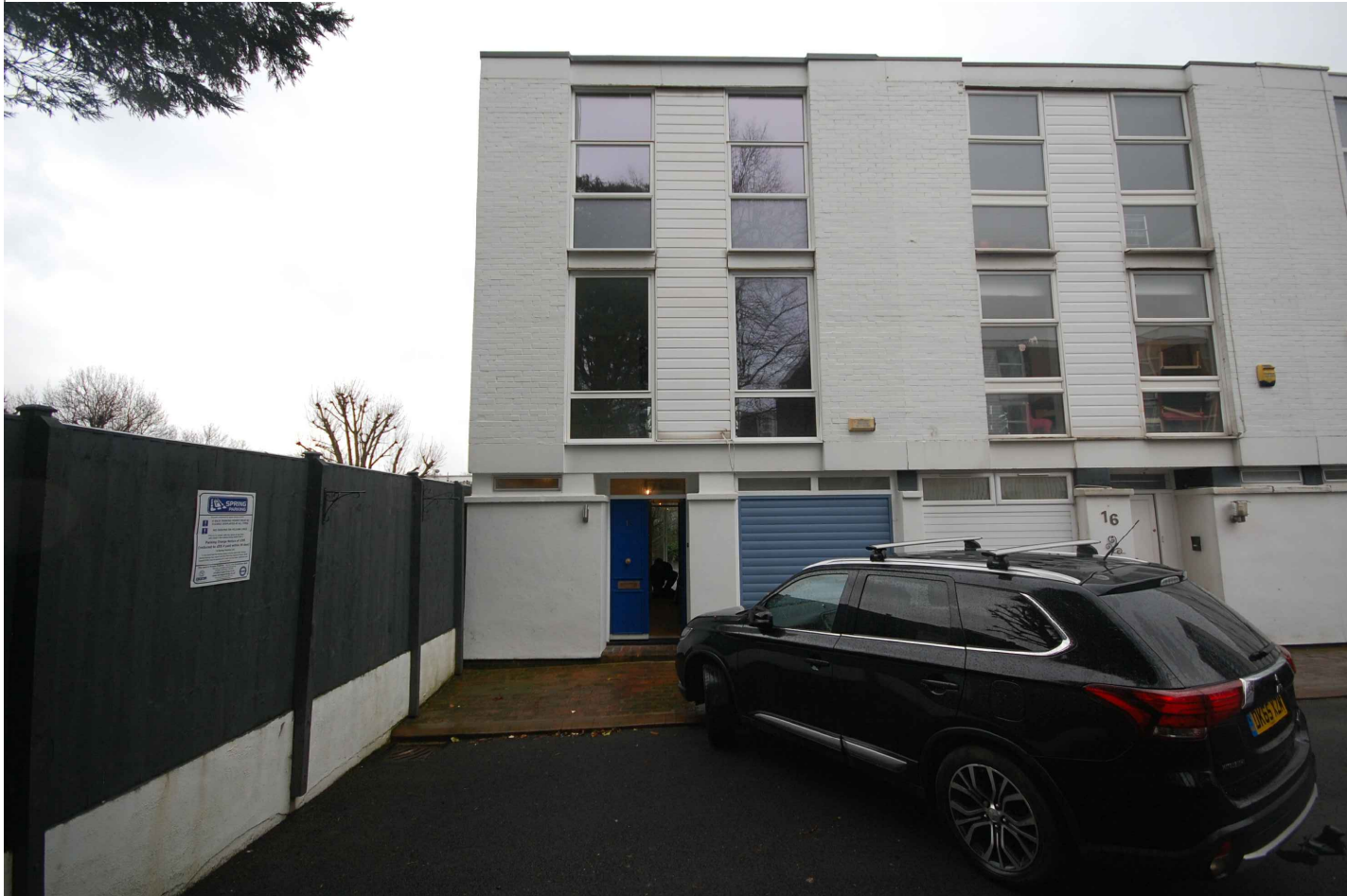
front elevation facing north
