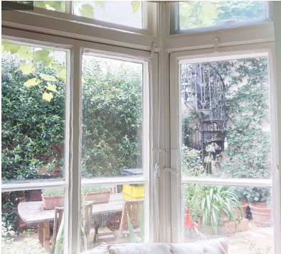
EXISTING NON-ORIGINAL CASEMENT WINDOWS IN POOR CONDITION.
