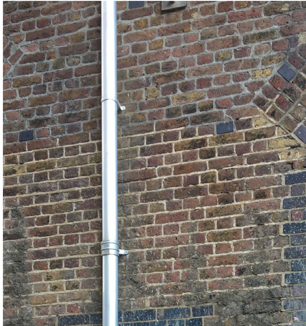
3. Existing Brickwork & galvanised downpipes
