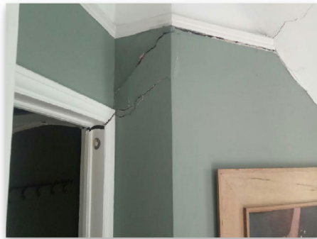
Fig 1.6: Internal cracking
