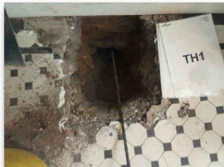
Fig 1.8: Trial Hole 2 Footing
