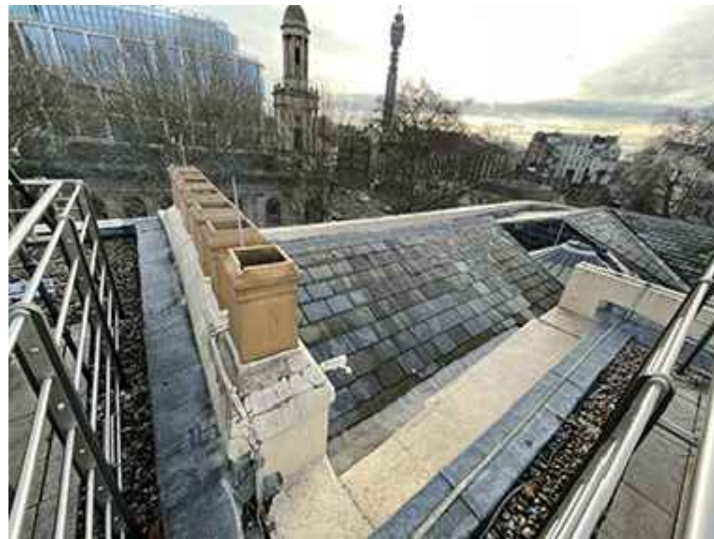
2 ROOF LOOKING EAST SCALE NTS
