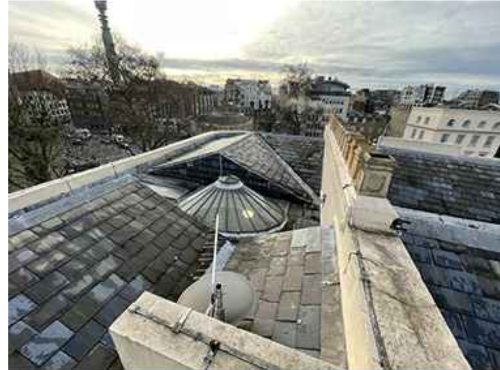
4 ROOF LOOKING EAST SCALE NTS
