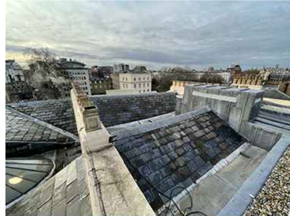
3 ROOF LOOKING EAST SCALE NTS
