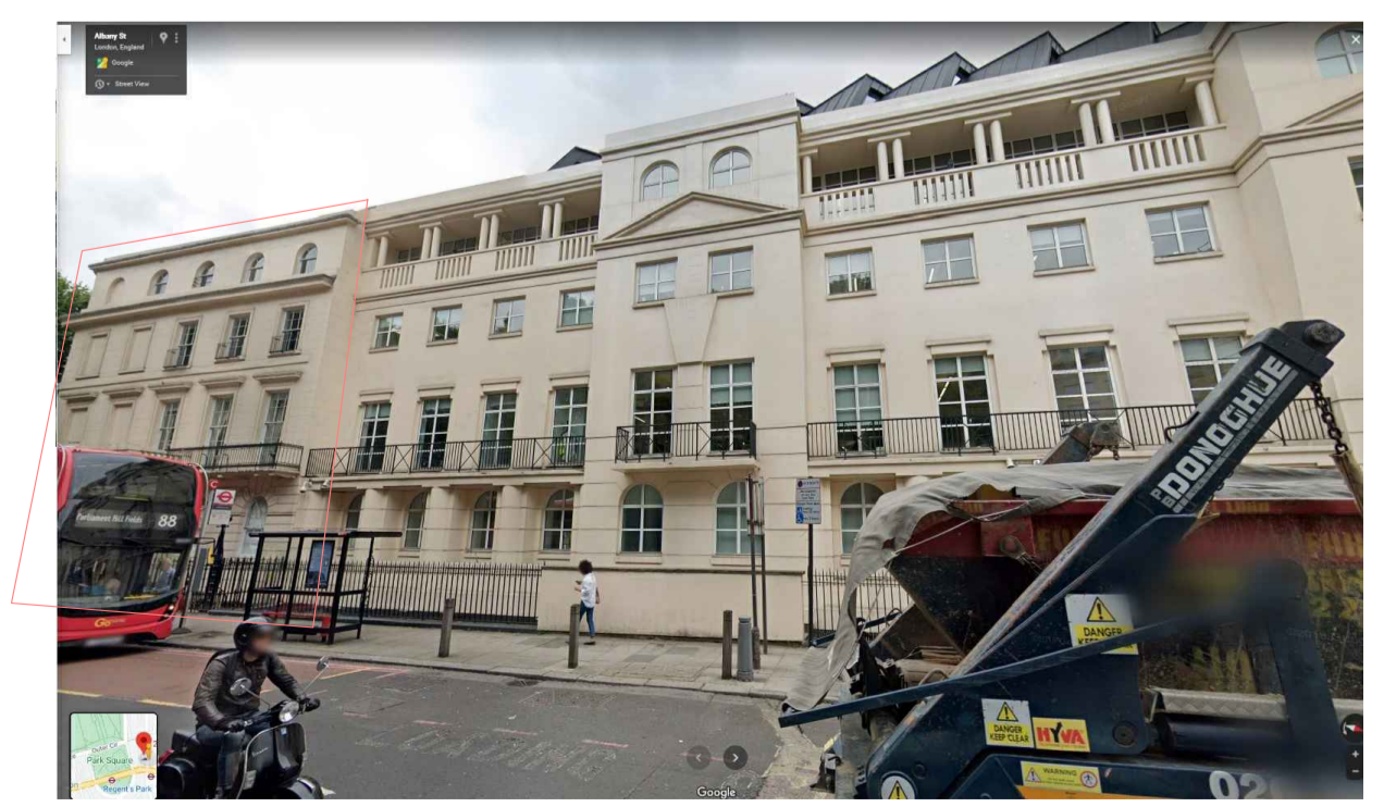
3 EAST SIDE FACADE TO GRADE 2 LIST BUILDING AND ADJOINING BUILDING SCALE NTS
