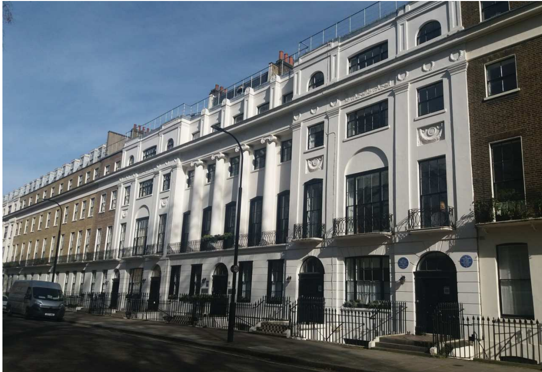
Context Oblique view of terrace centre pavilion stucco facade – looking north – starting with No. 21 on right with existing two plaques
