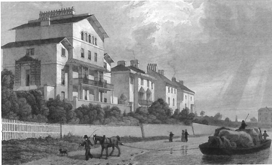
Figure 8: 'Park Village East, from the Regent's Canal. In the foreground are the rear elevations of nos. 6-8. Drawing by Thomas H Shepherd, c.1829', in The Camden Town Book, John Richardson (London, 2007), p. 100.
