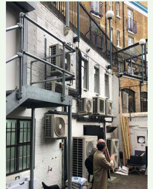
EXISTING CONDENSER UNITS TO THE REAR OF THE COURTYARD AND ROOF.
