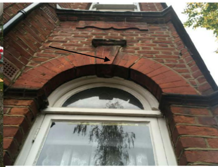
Crack to brick arch
