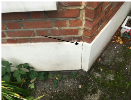
Vertical crack to left side junction of bay
