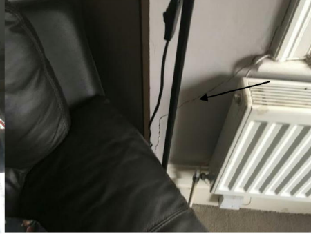
Front lounge – diagonal crack to right side bay
