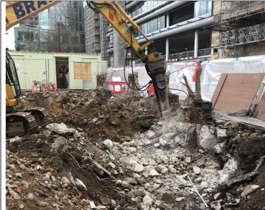
Photo 5 Image facing south-east showing obstruction (concrete piles) removal.
