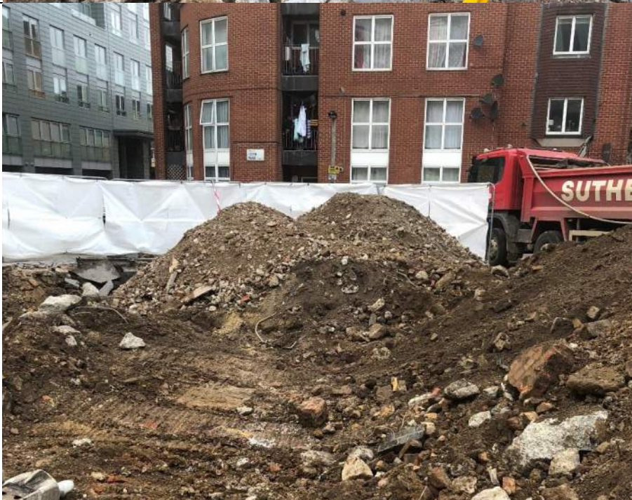
Photo 2 Image facing west showing stockpile of imported material used to raise levels to support excavator.
