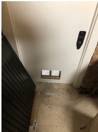
Figure 2: Existing ventilation grate in lightwell door
