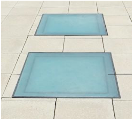
GlazingVision walk-on rooflight to replace existing. Etched glass for privacy, laminated glass for safety. Flush with pavement.
