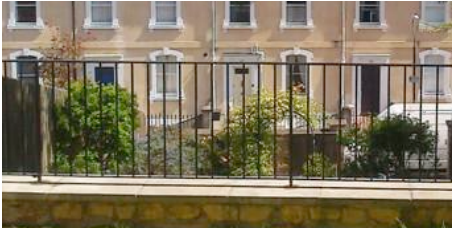
Plain wrought iron railings by the London Metal Fabrications. 40 x 8mm rails to top and bottom, 12mm vertical bars 98mm apart. Painted black.
