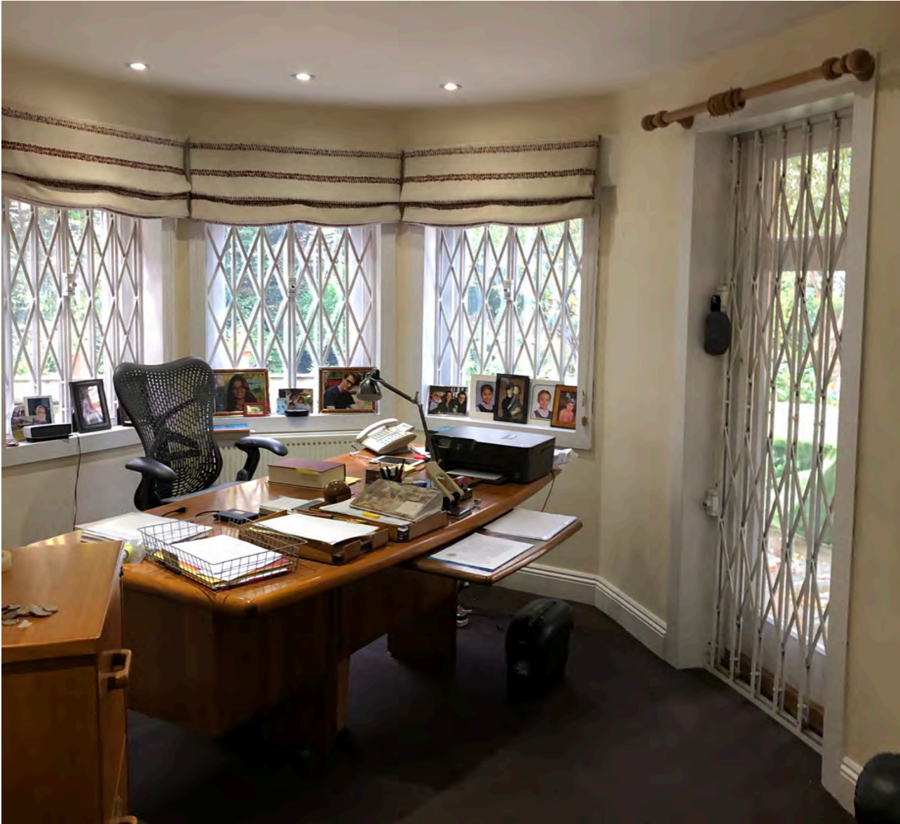
Figure 11: Internal view of the three office windows and glazed door at basement
