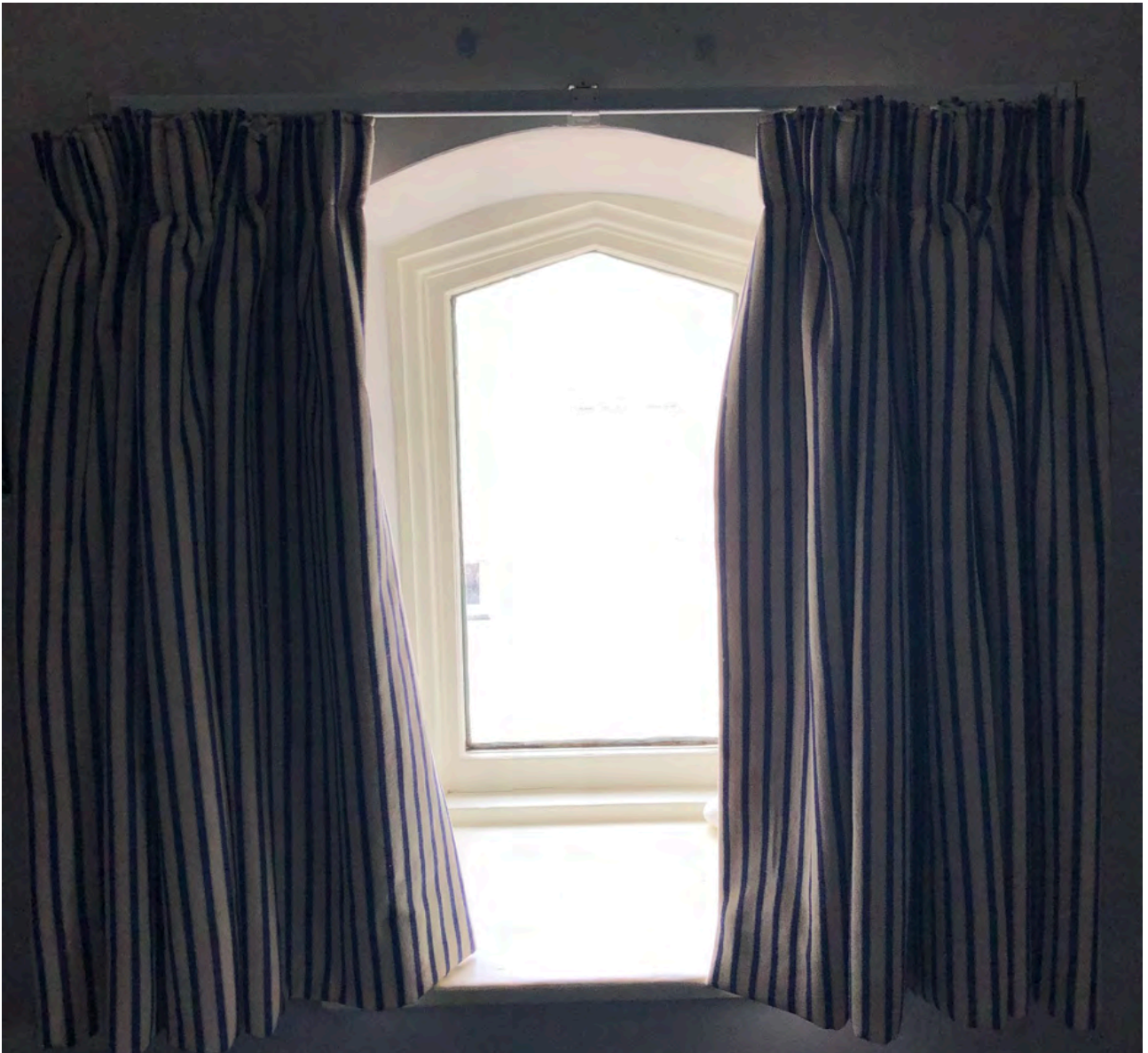
Figure 20: Internal view of window in bedroom A at second floor
