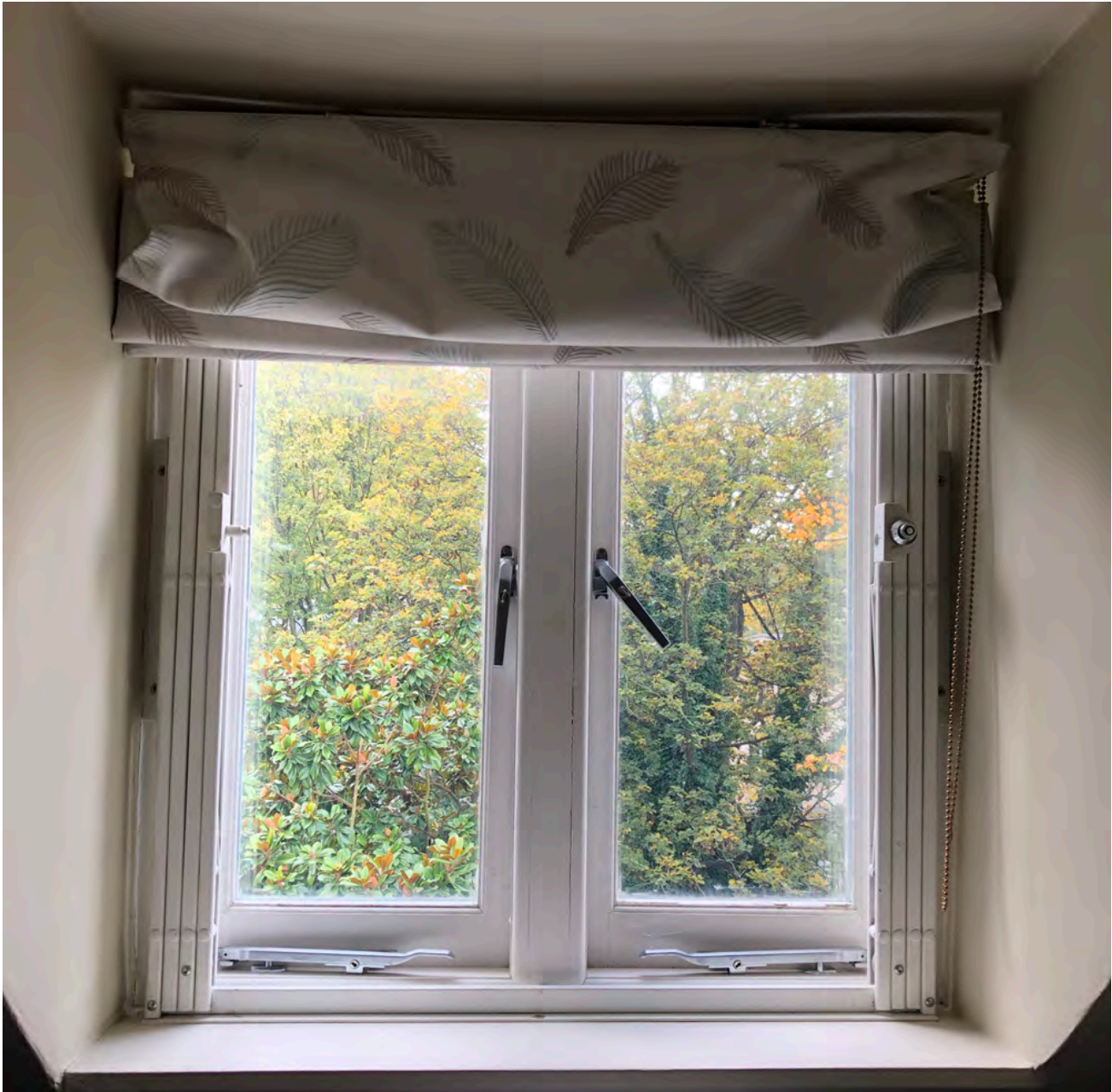
Figure 22: Internal view of window in bedroom B at second floor
