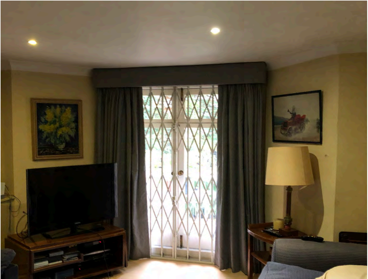
Figure 10: Internal view of patio door in the lounge at basement
