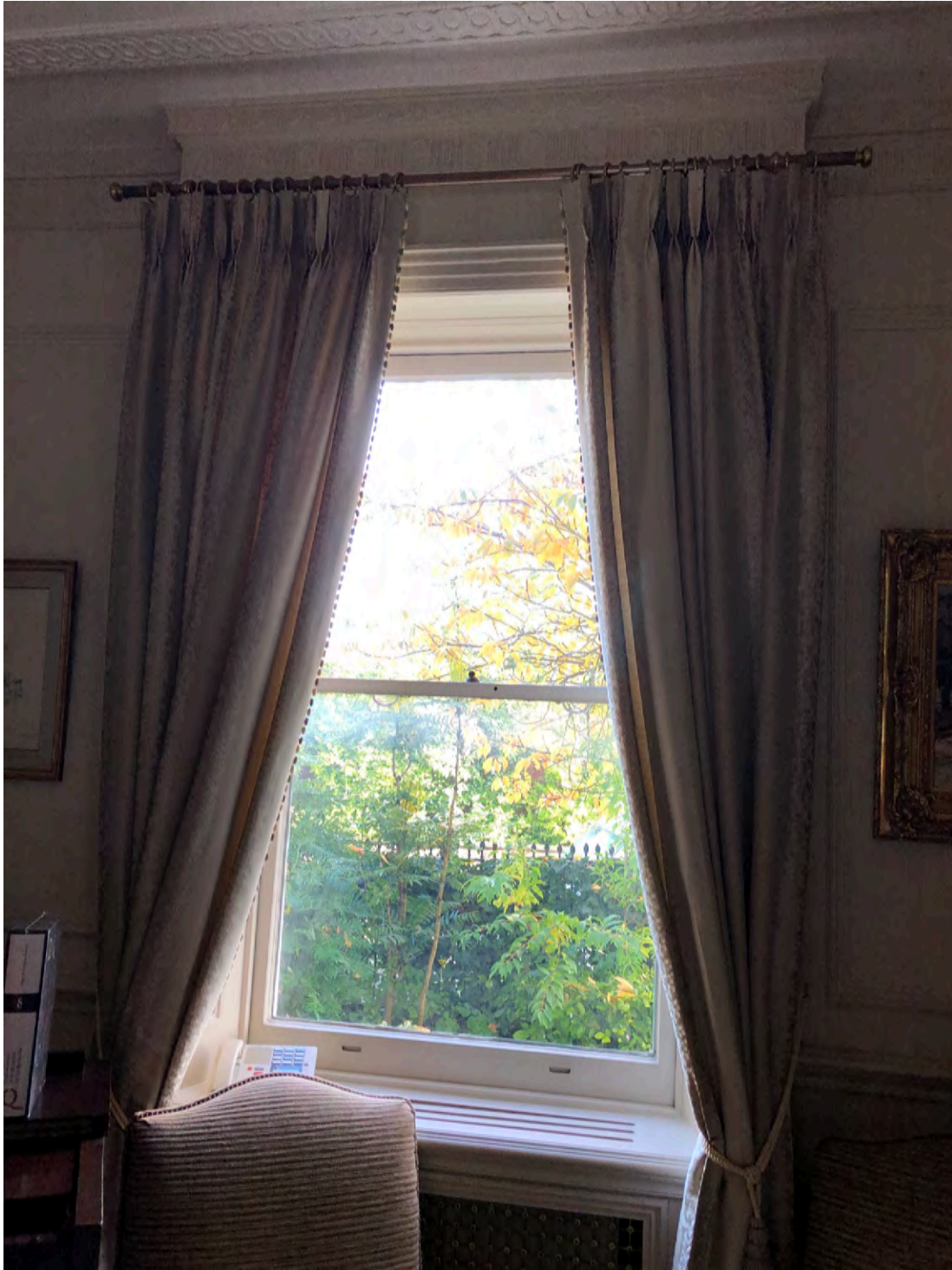
Figure 14: Internal view of the right-hand side window in the lounge at ground floor level
