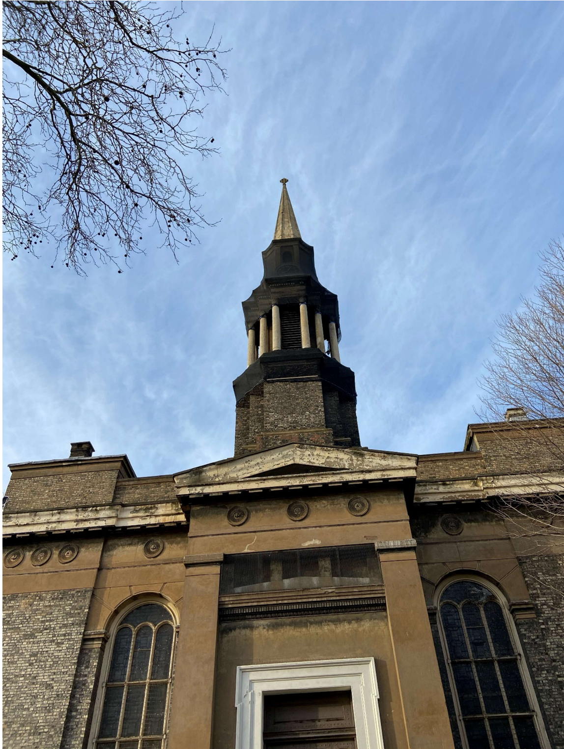
Img. 3; Black netting installed to tower
