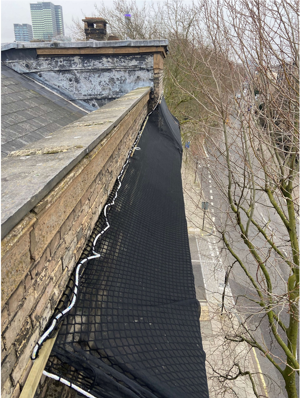
Img. 2; Close-up view of black netting installed to sky-facing edge of cornice
