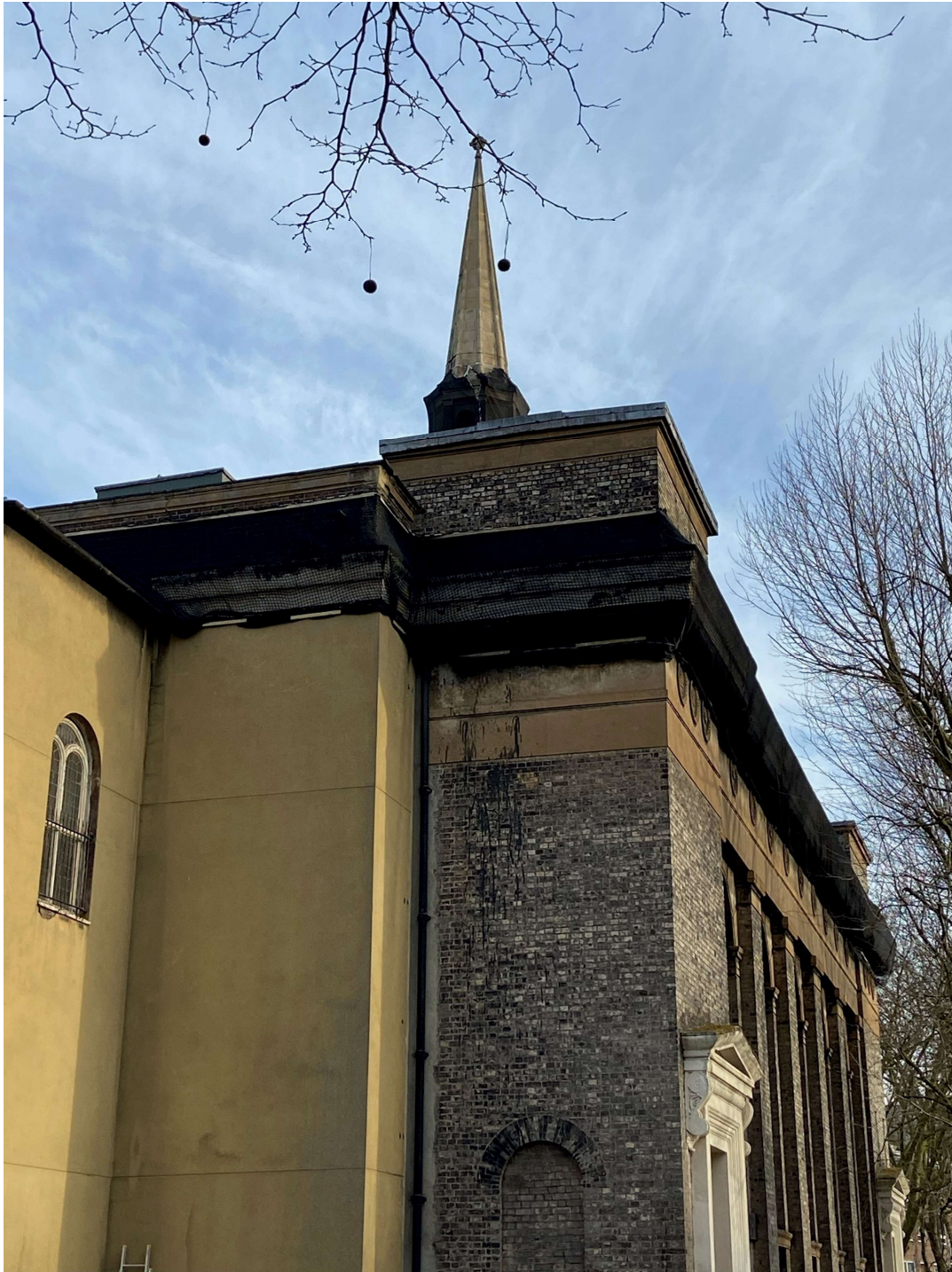
Img. 1; Netting installed to the cornice
