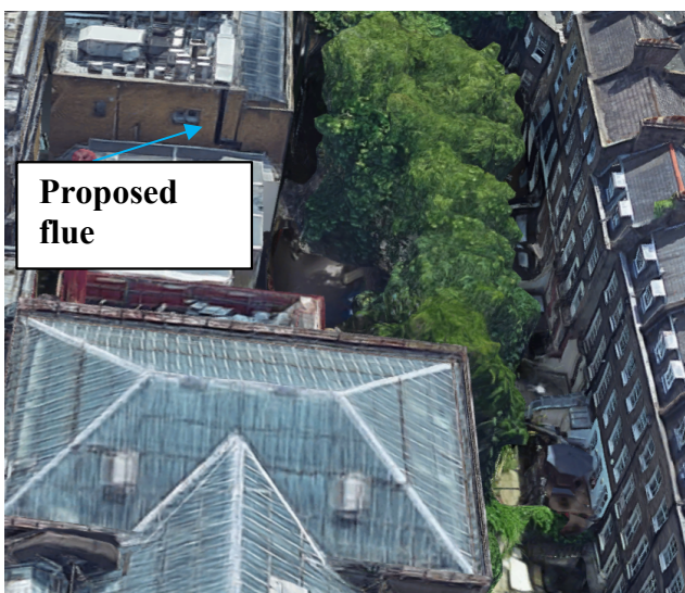
Figure 1 View of the extract flue
