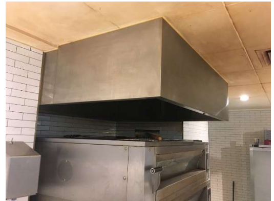
Figure 01, Existing oven and canopy
