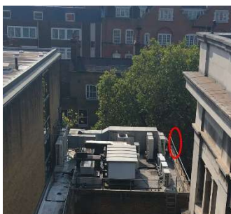
Figure 2, Western View point over existing kitchen plant and flue terminal indicator
