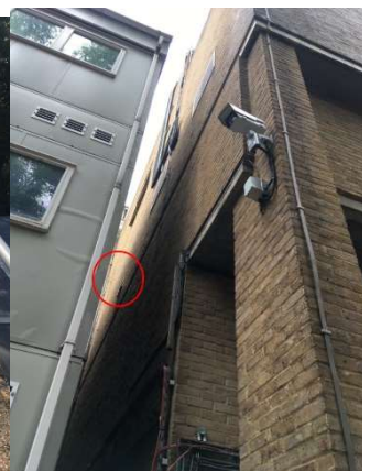
Figure 5, Vent stack exit point to external from ground level perspective
