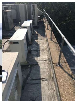
Figure 4, Vent stack to terminate 1m above the edge parapet, behind the edge protection.
