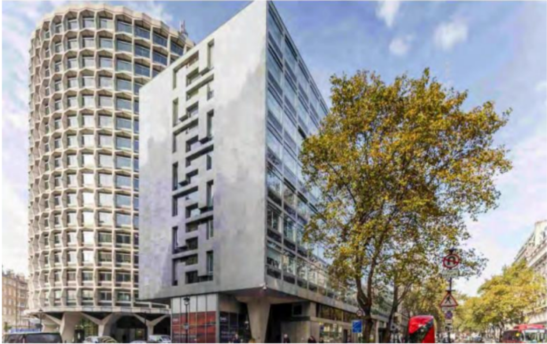
Figure 1: The existing site viewed from Kingsway
