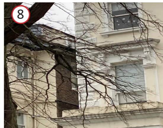
24 Belsize Park 4 casement windows
