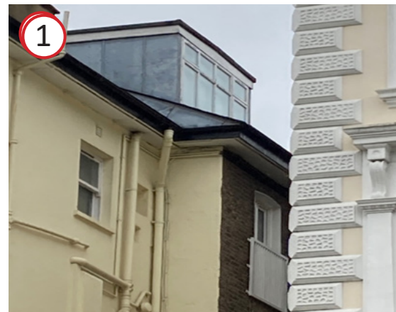
34 Belsize Park 4 casement windows with fanlight over
