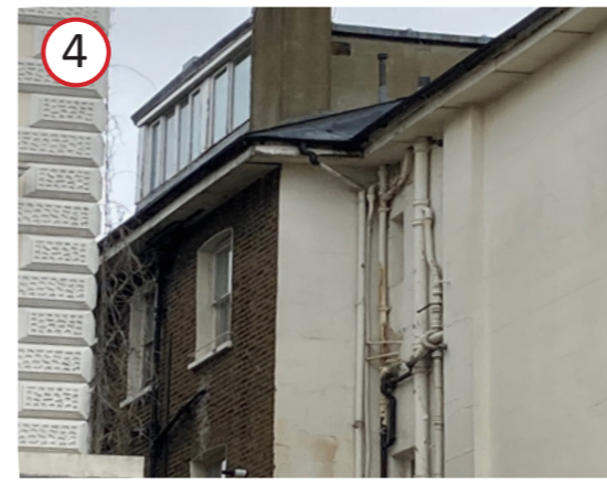
31 Belsize Park 6 casement windows
