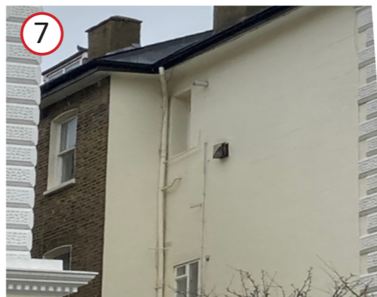
25 Belsize Park 2 casement windows
