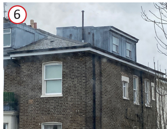
29 Belsize Park 2 sash windows with large side panels
