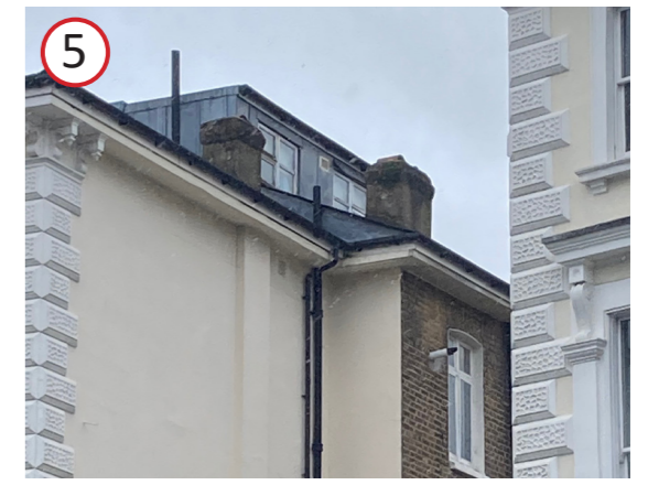
30 Belsize Park 4 casement windows with large side panels
