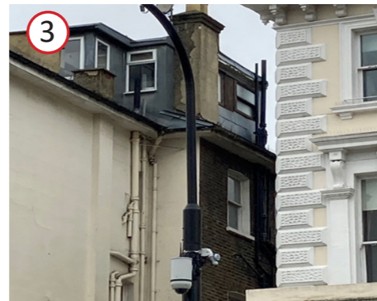
32 Belsize Park 2 casement windows with large side panels
