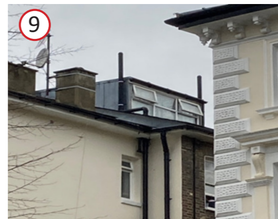
20 Belsize Park 3 casement windows
