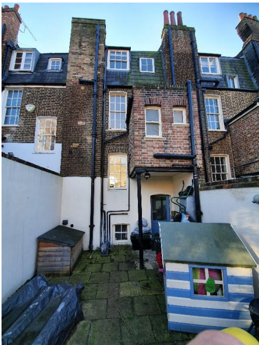
Rear elevation of 27 Jeffreys Street
