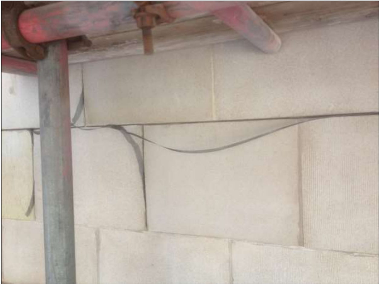
Photograph 1 – Anode ribbon prior to grouting into the masonry joints.
