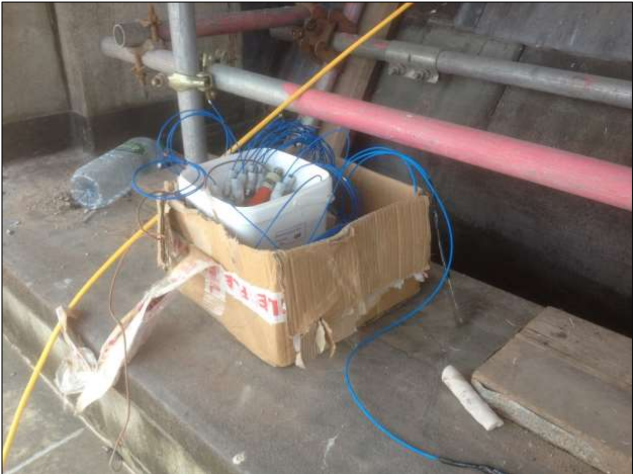
Photograph 2 – A set of reference electrodes on site ready for installation
