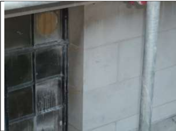
Photograph 9 – Re-pointed stonework after CP installation
