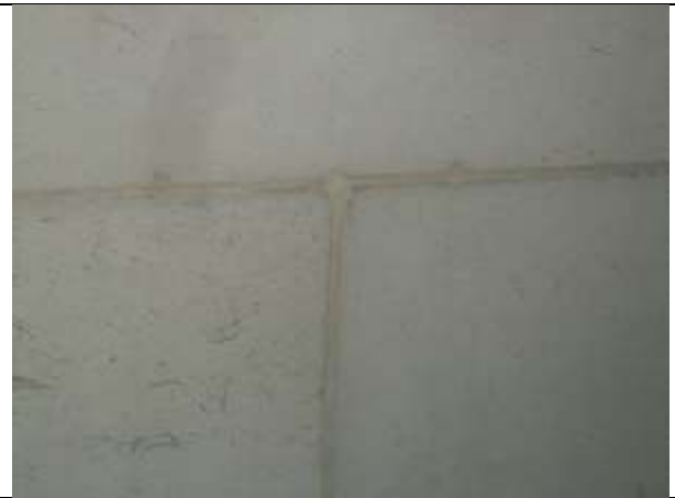
Photograph 10 – a close-up view of repaired/re-pointed stonework.
